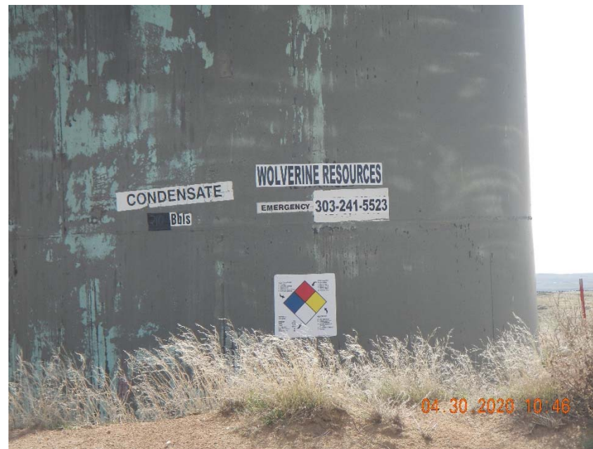
Photo 4. No flammability numbers on NFPA diamond.
