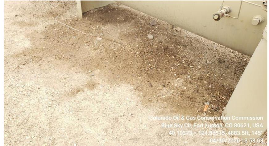
**Photo 7 Stained soil by Horiz. Heated Sep.**
