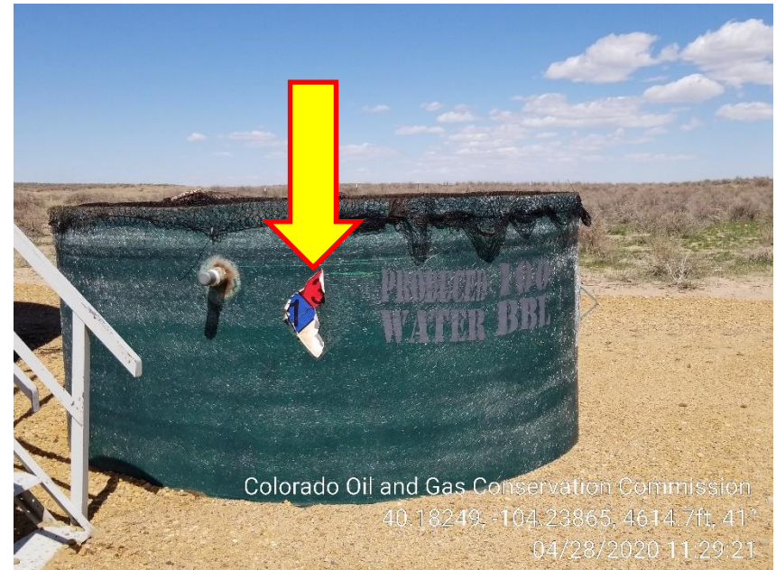
Photo 4 – Produced Water, NFPA Label is peeling/fading
