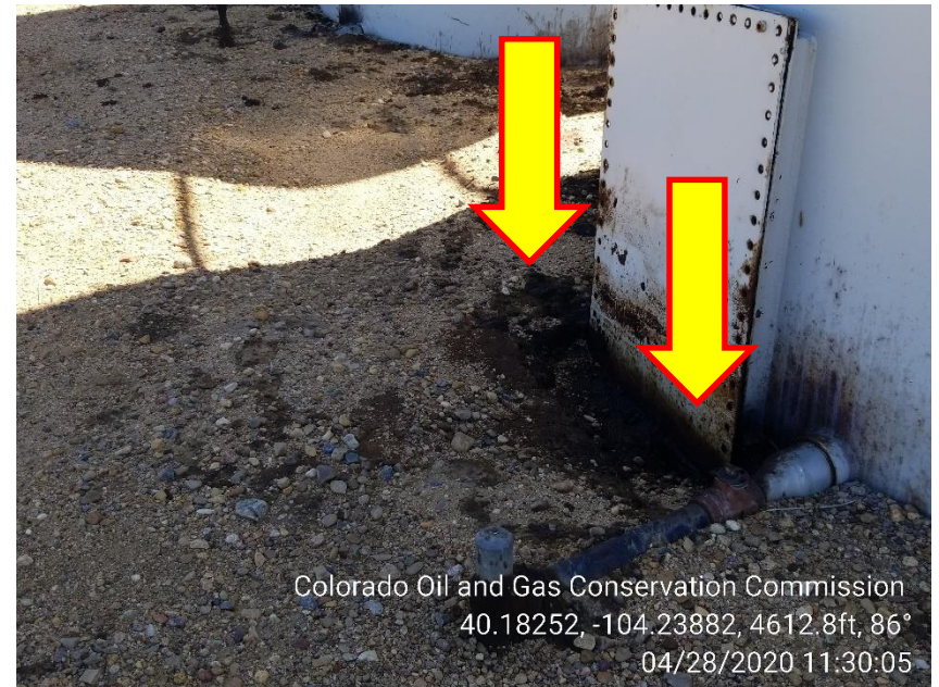
Photo 8 – Stained Soil at cleaned out plate on West Tank
