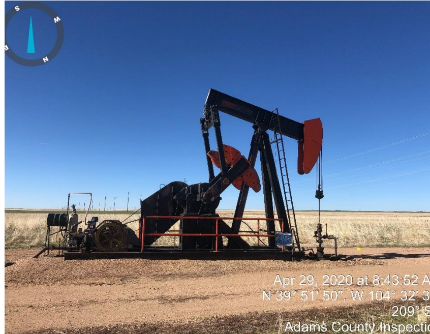
Photo #1 pump jack
