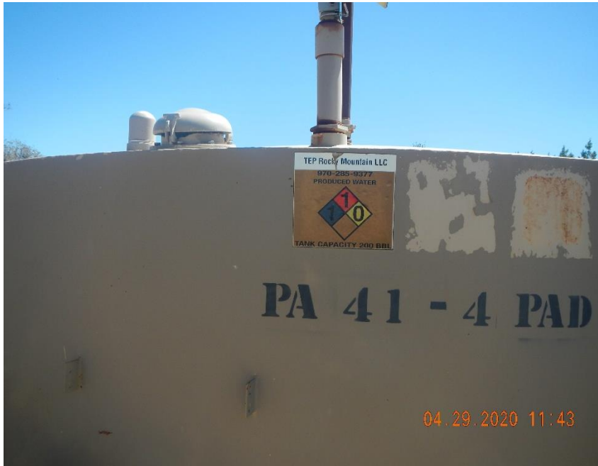
Tank labels are discoloring and peeling.
