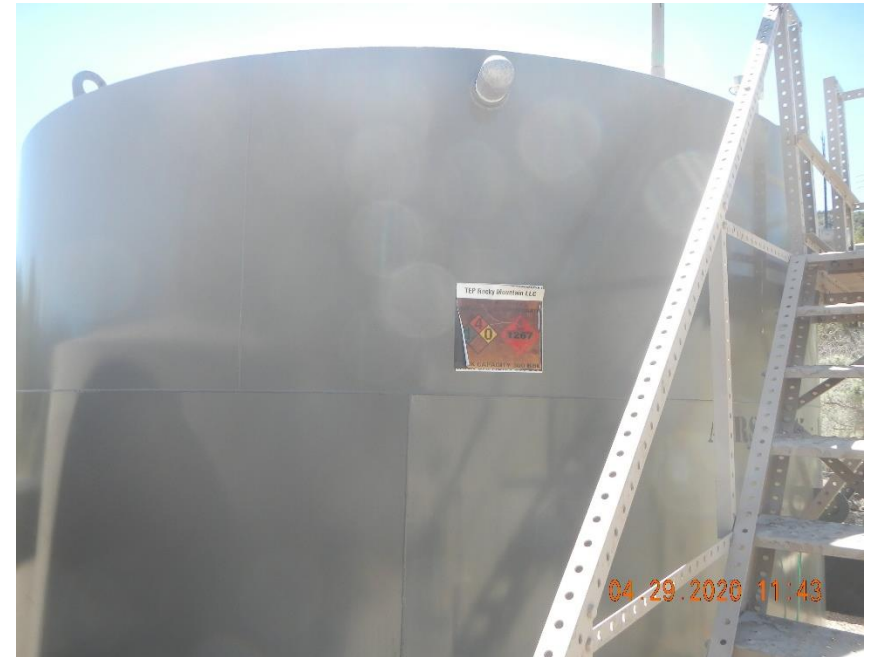
Tank labels are discoloring and peeling.
