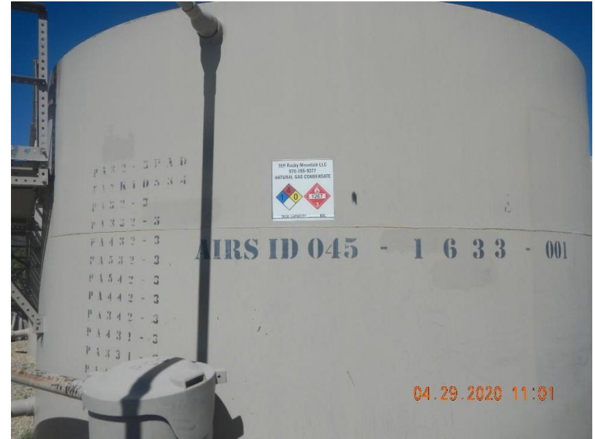
Tank capacities are faded / inadequate size font.
