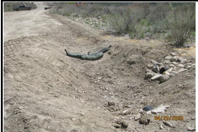
Sediment Trap & Flex Pipe Outlet on the West Side of the C.C. 629-23-42 Pad
