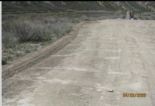
Grading and Berm Installation on the West Side of the C.C. 629-23-42 Pad
