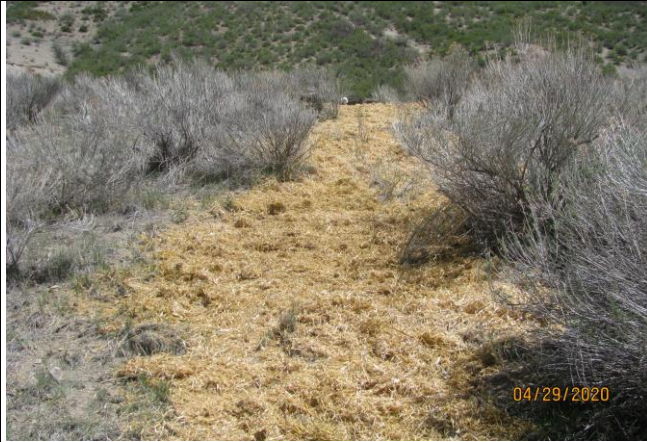
Disturbance Broadcast Seeded & Mulched on the C.C. 629-23-42 Fill Slope
