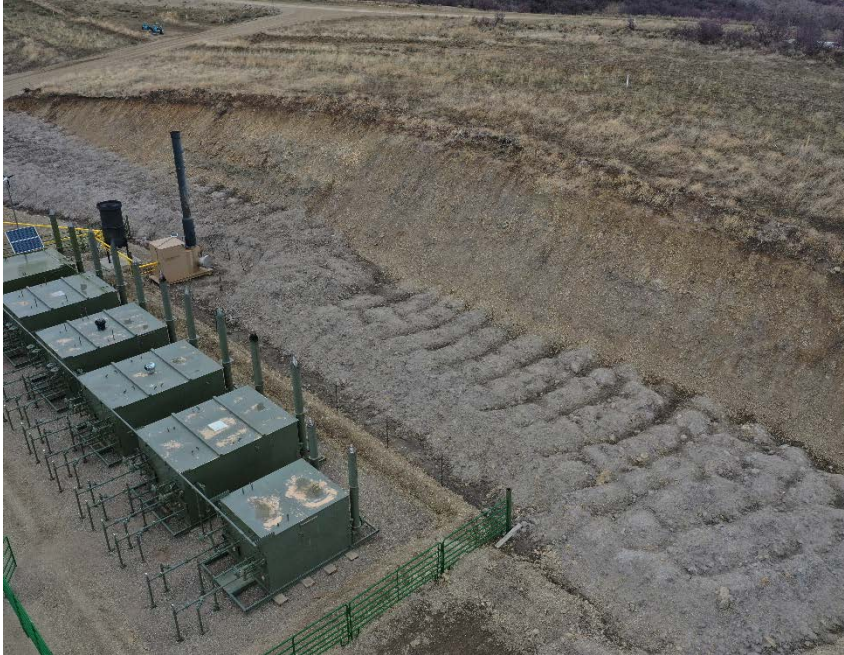
Photo #5 – Aerial view of cut slope on east side of pad. Beneficial reuse of cuttings described in doc #402163214 has not been completed.
