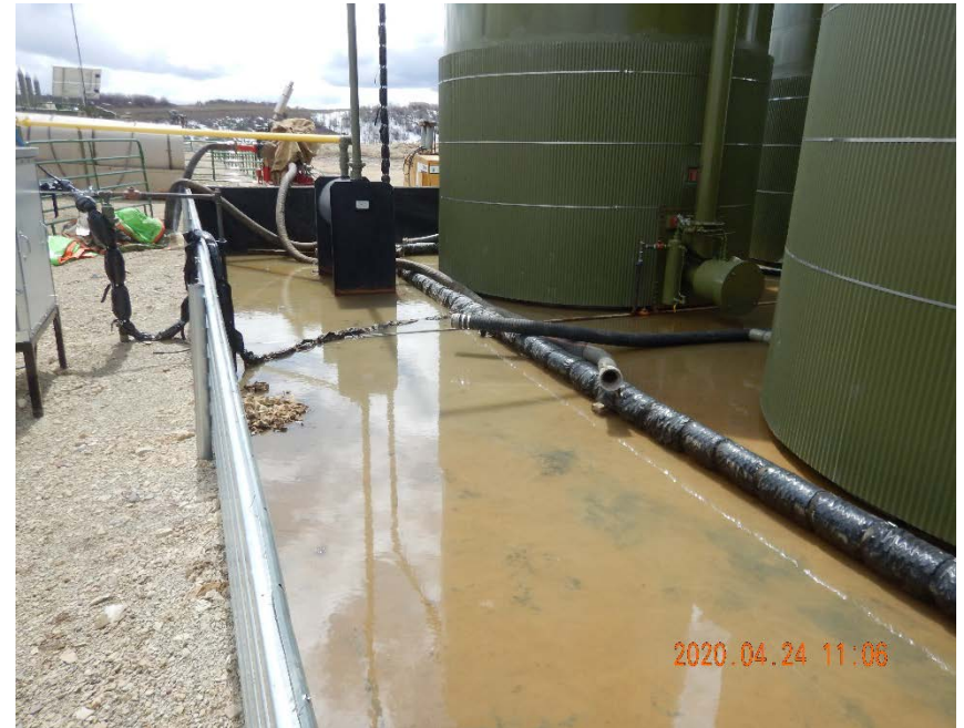
Photo #2 – View of fluids inside of tank battery secondary containment area (east side). Note hoses stored inside of secondary containment area.
