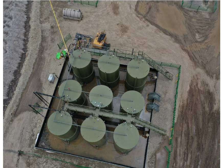
Photo #4 – Aerial photograph of tank battery documents the amount of fluids present in secondary containment area during inspection.
