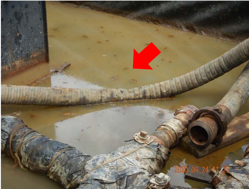
Photo #3 – Mixed fluids, hoses with metal fittings, and wood debris inside of tank battery secondary containment area (SE corner). Note presence of condensate floating on fluids (red arrow). Hydrocarbon odors were observed in this area.
