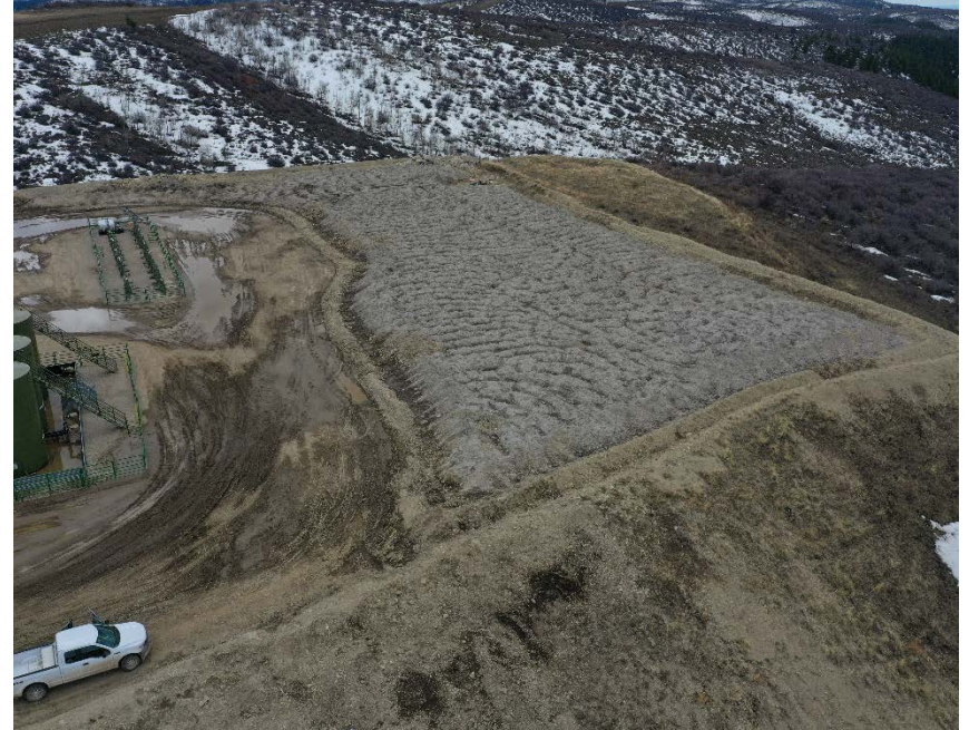
Photo #6 –Overview of land treatment area in southwest side of pad. Land treatment of cuttings is documented under Remediation Project #11653, which was approved for closure on 10/9/2018 (doc #401752256).
