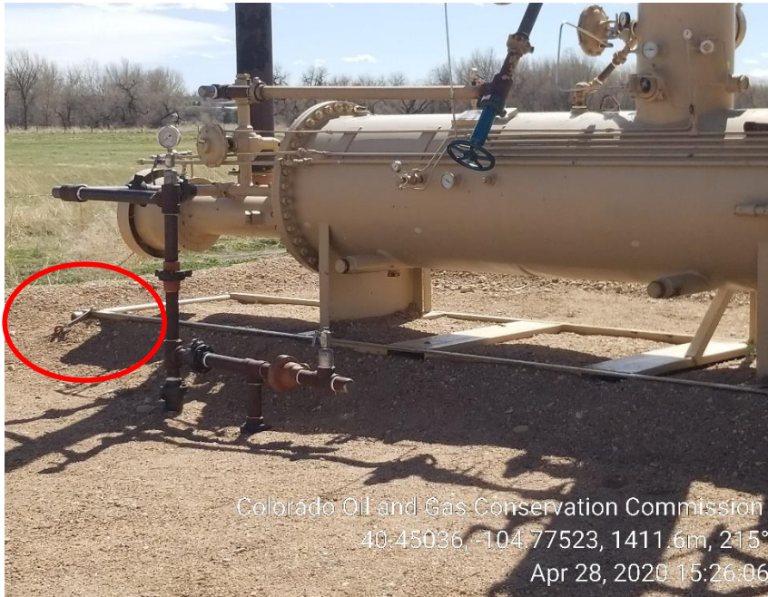
Photo 3: Separator anchored
