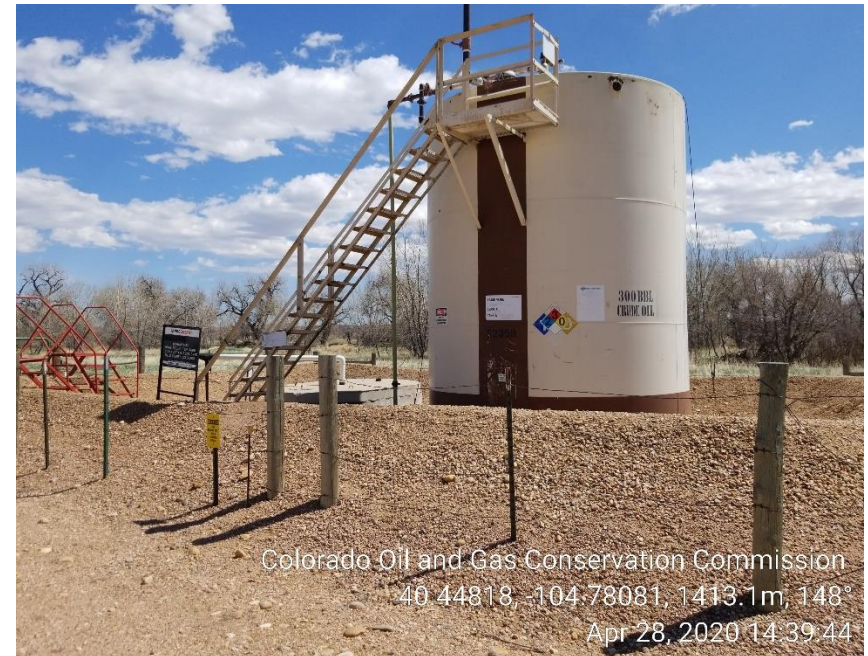
Photo 4: Tank Battery; inadequate berm
