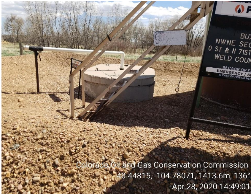
Photo 5: H2O tank not anchored.
