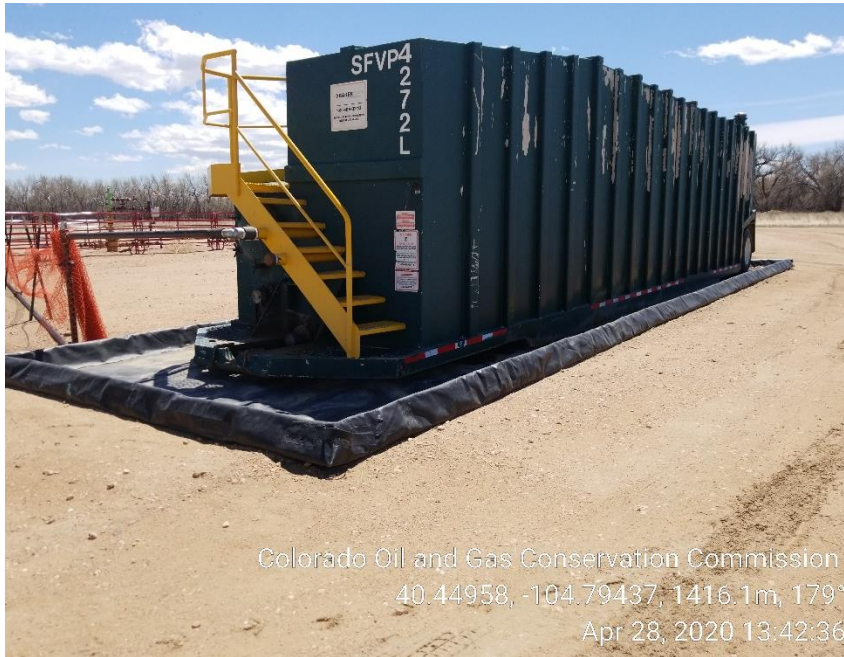
Photo 25: Tank not grounded
