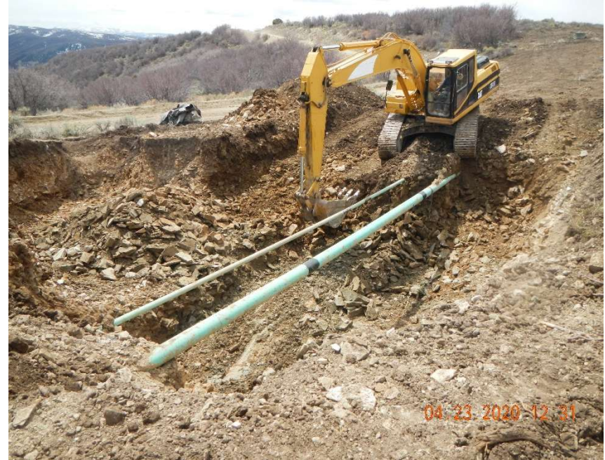
View of the excavation, 4-inch and 8-inch pipeline
