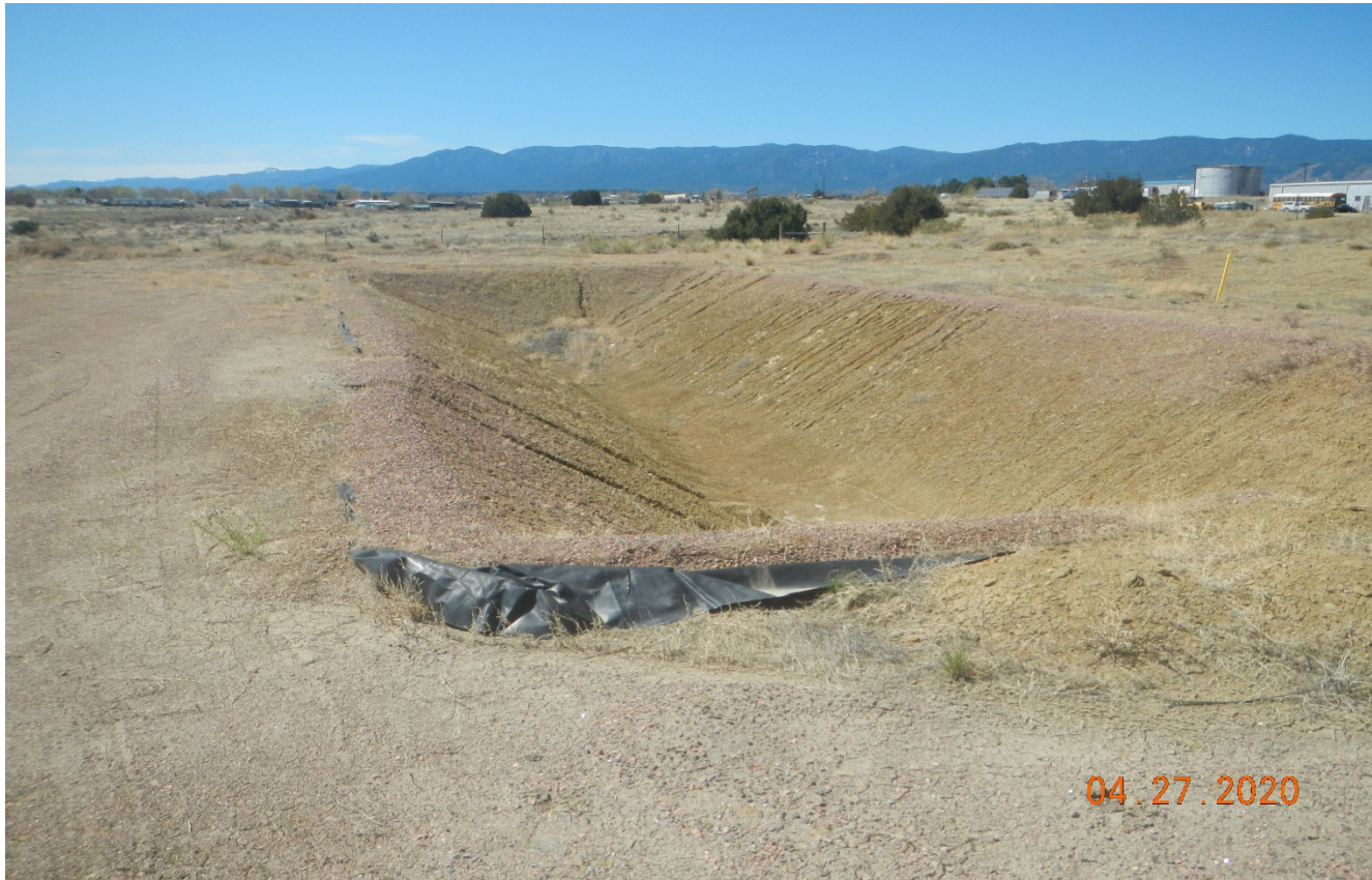
Photo 5. The pit has not been closed and reclaimed as required.
