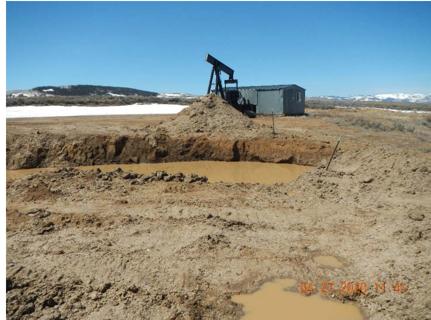
Photo 4. Pump jack and excavation work remain on location and incomplete.
