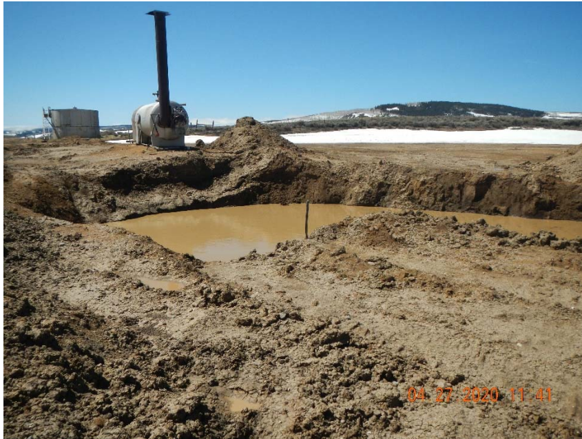
Photo 3. Separation equipment and excavation work remain on location and incomplete.
