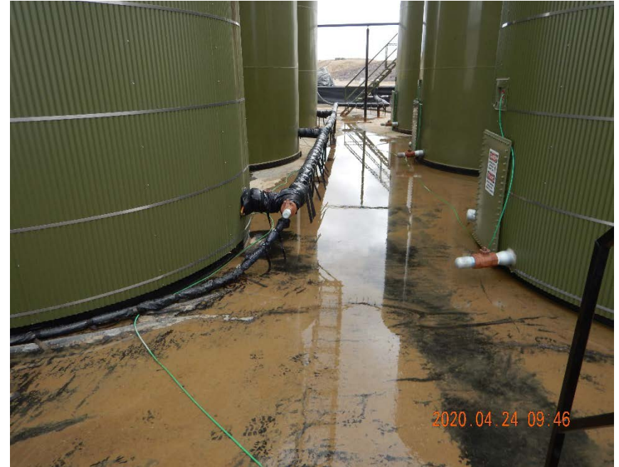
Photo #6 – Localized accumulation of fluids inside of tank battery secondary containment area.
