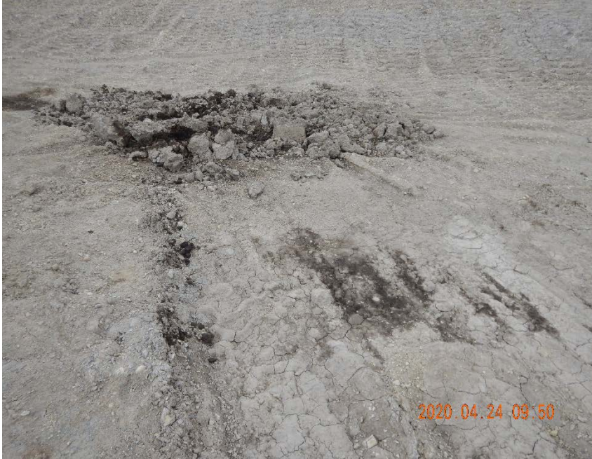
Photo #11 - Localized accumulation of oil-stained soil on west side of pad. (4)
