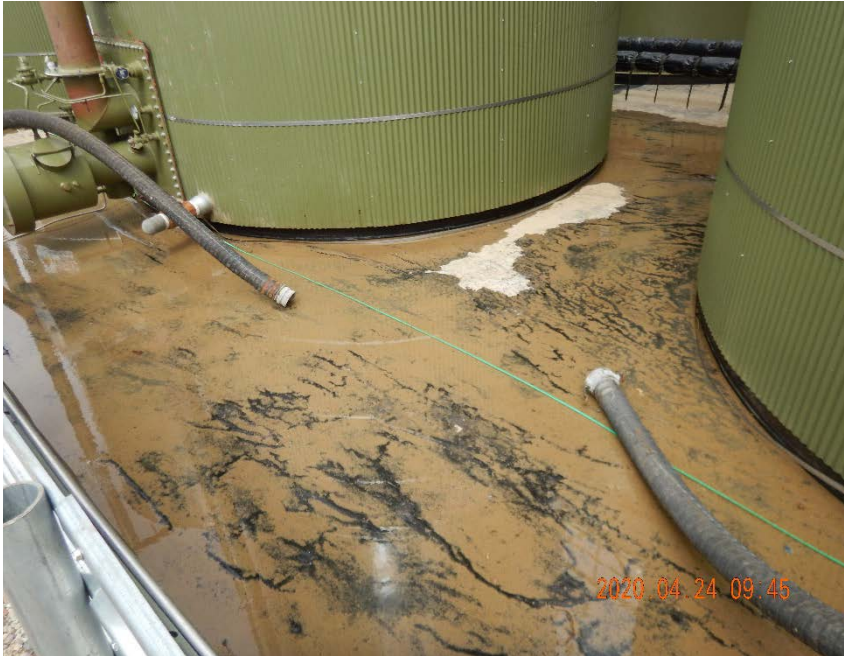
Photo #5 – Localized accumulation of fluids inside of tank battery secondary containment area. Note storage of hoses in secondary containment area with metal fittings in direct contact with liner.
