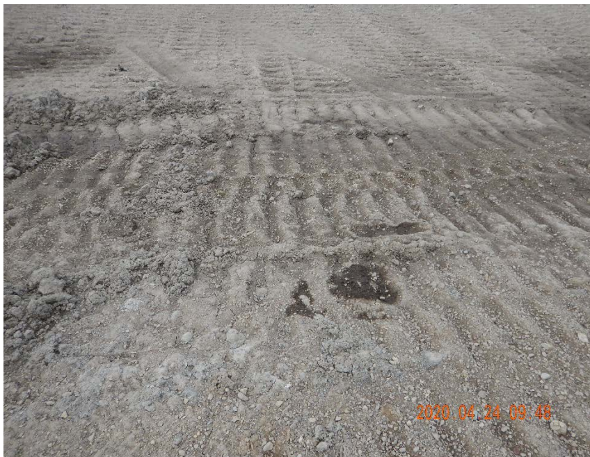
Photo #9 - Localized accumulation of oil-stained soil on west side of pad. (2)
