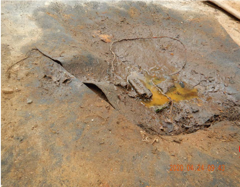
Photo #3 – Hole observed in tank battery liner on east side, beneath loadout area. Operator was contacted via phone on 4/24/2020 and instructed to repair liner.
