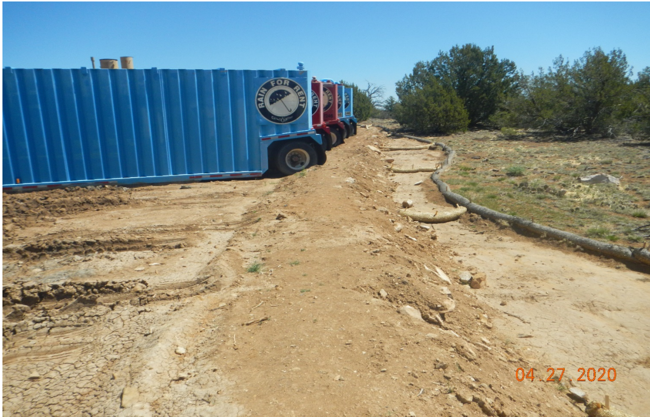
Photo 6. This berm along the backside needs to be leveled and recontoured for interim reclamation. There are wattles placed along the backside of the berm.
