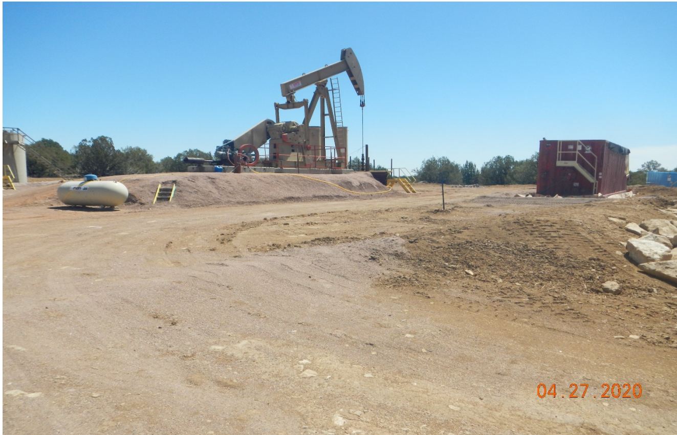
Photo 13. The northwest side of the location has been stabilized with rock rip/rap.
