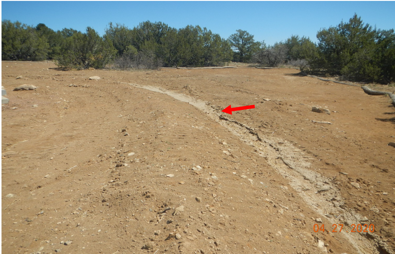
Photo 8. Facing toward the northeast area of the location. This area needs to be seeded and reclaimed. Additional BMP's may be needed along the stormwater diversion shown by red arrow.
