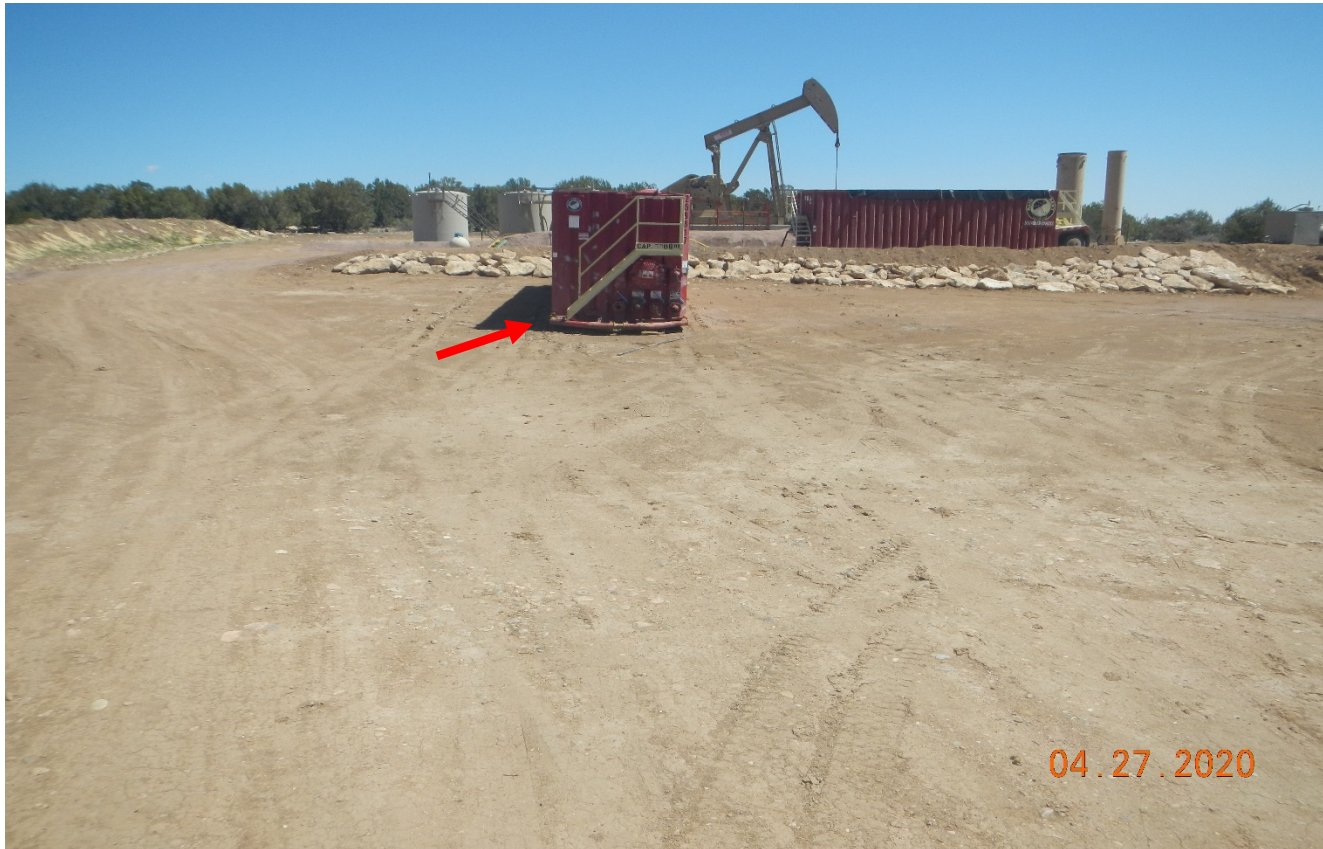
Photo 3. Facing north toward the location. This red tank shown by arrow has not been removed and this area has not been reclaimed. Previous corrective actions have not been performed.
