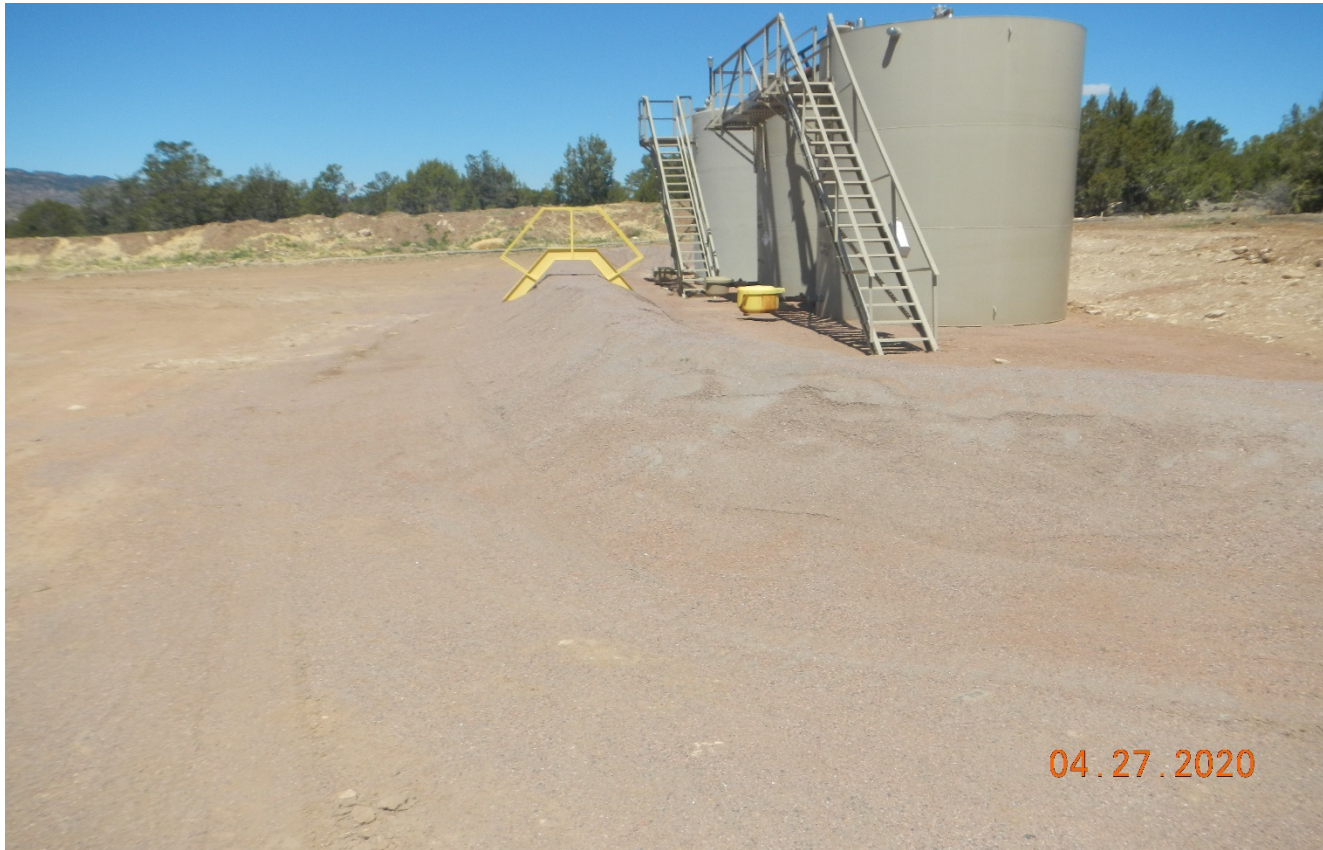
Photo 9. The berm around the tank battery has been compacted.
