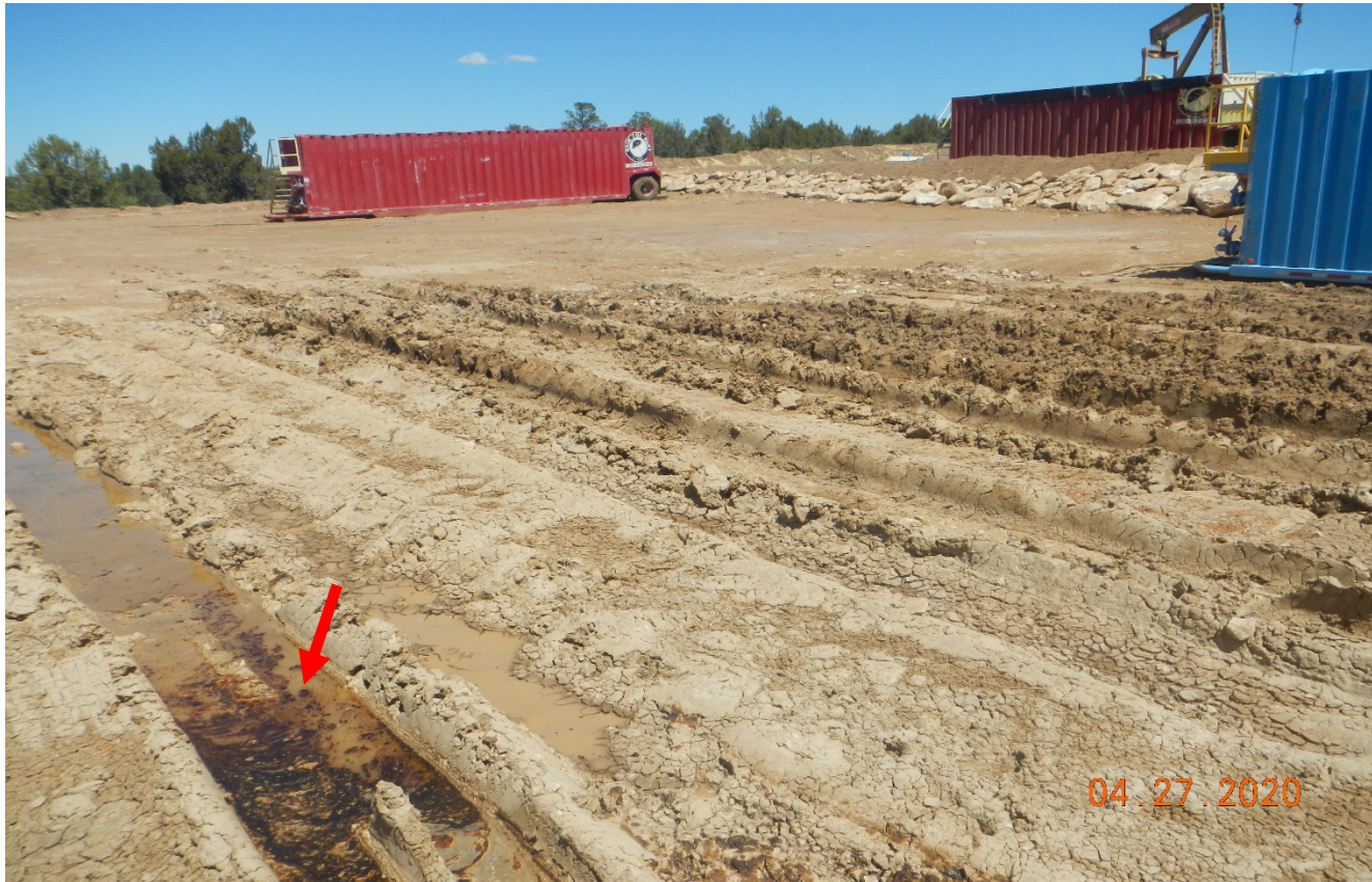
Photo 5. Facing northwest where tanks had been stored. There is deep vehicle rutting in this area which will create pooling of water. There is oily water in the ruts shown at red arrow. This area needs to be recontoured and reclaimed.
