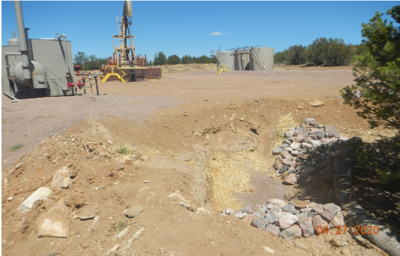
Photo 7. Facing northwest toward the well site. There is a sediment trap at this east side of the location.
