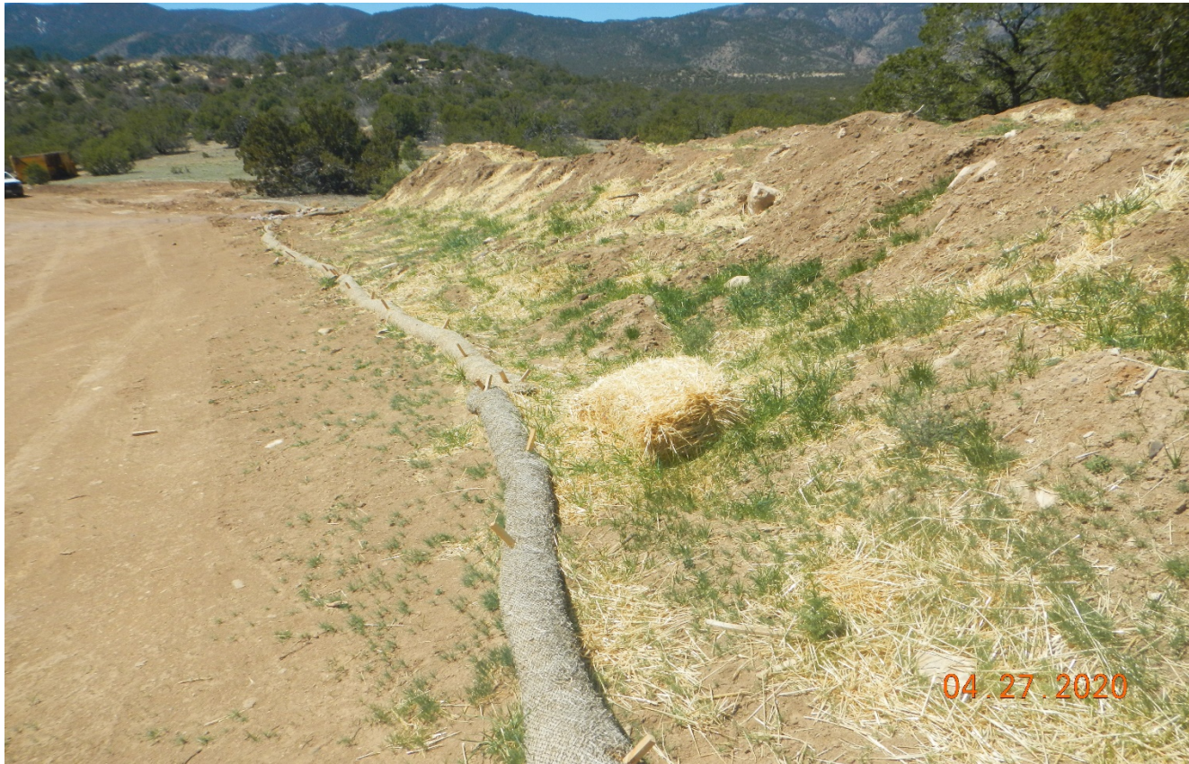
Photo 10. The wattles have been repaired along the topsoil pile. It appears the pile has been seed however, the topsoil pile should have been sloped and stabilized. There were weeds observed growing along the soil pile.
