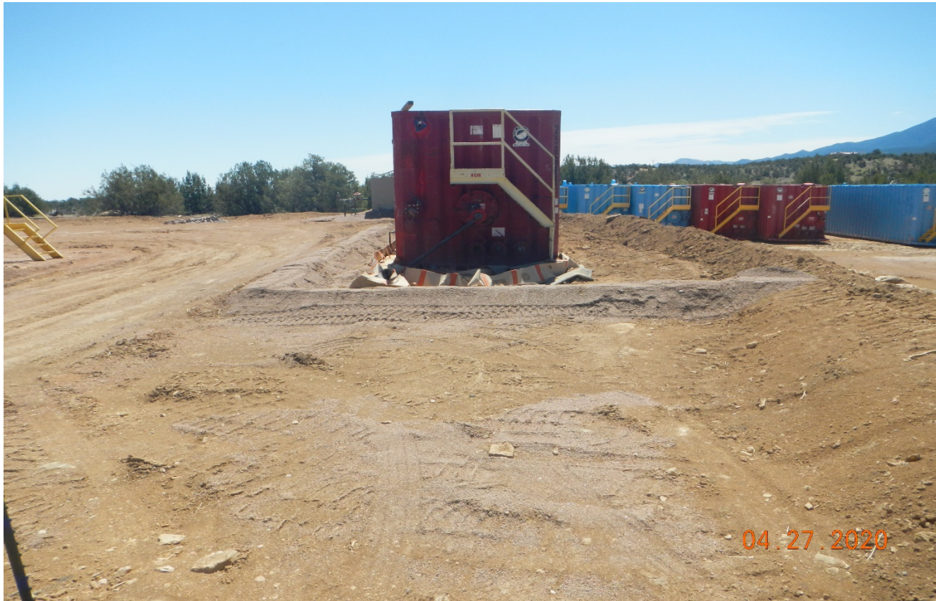
Photo 14. A compacted berm has been installed at the tank which appears to be in use.
