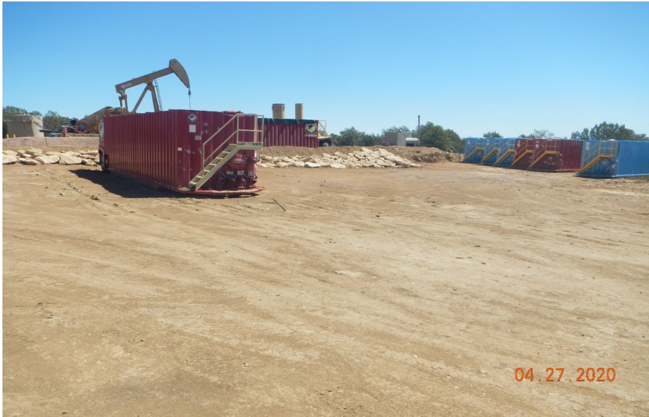
Photo 16. Facing northwest toward the location. The unused tanks need to be removed. This area needs to be recontoured and reclaimed. Previous corrective actions have not been performed.
