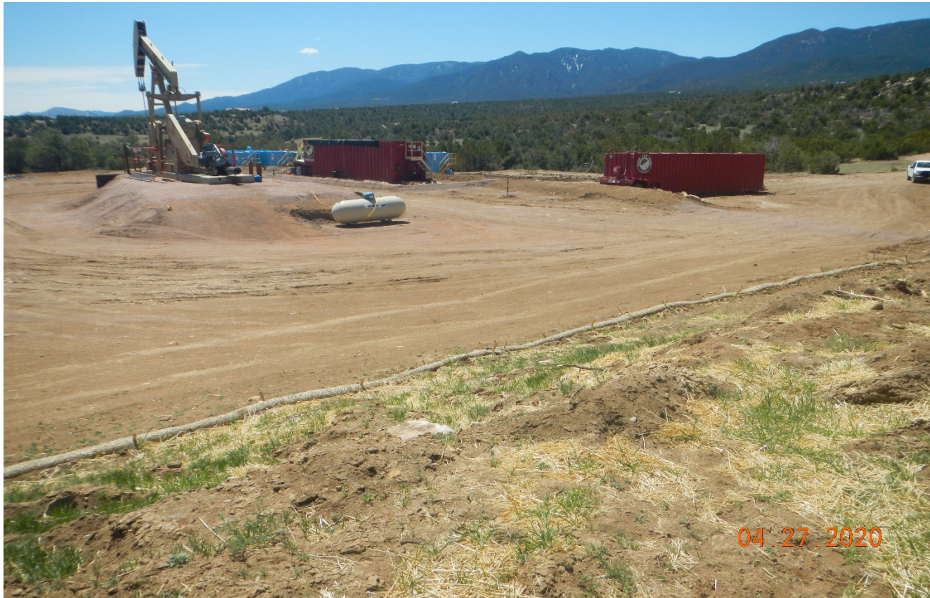
Photo 12. Facing southwest toward the location. A portion of the topsoil pile will need to be utilized for interim reclamation in the area where the frac tanks remain.
