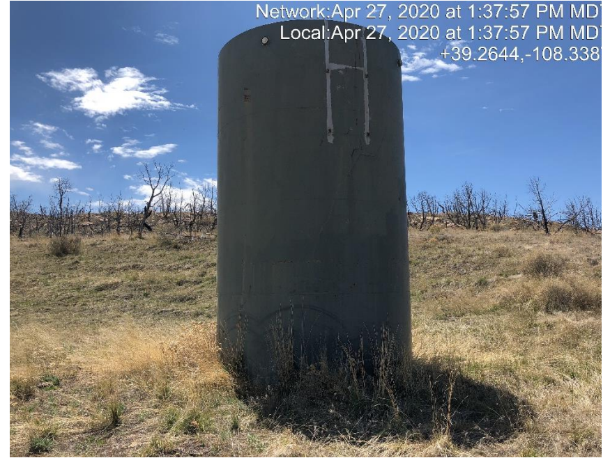
Photo #1068 Tank has been disconnected.
