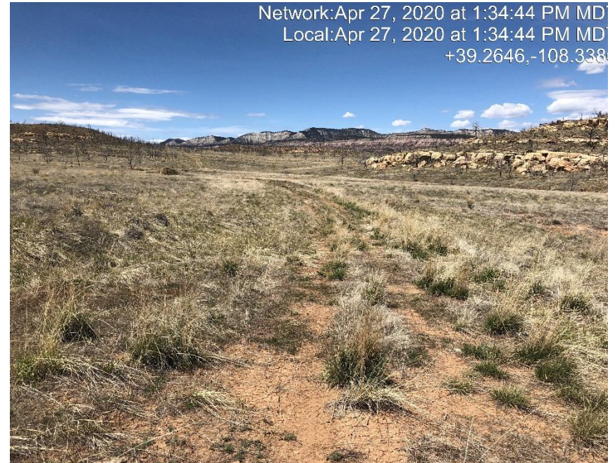
Photo #1061 Lease road has not been maintained.
