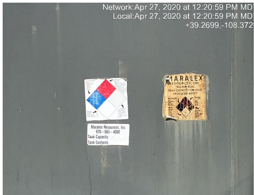
Photo #1053 Tank capacity, contents and NFPA label weathered and not legible.
