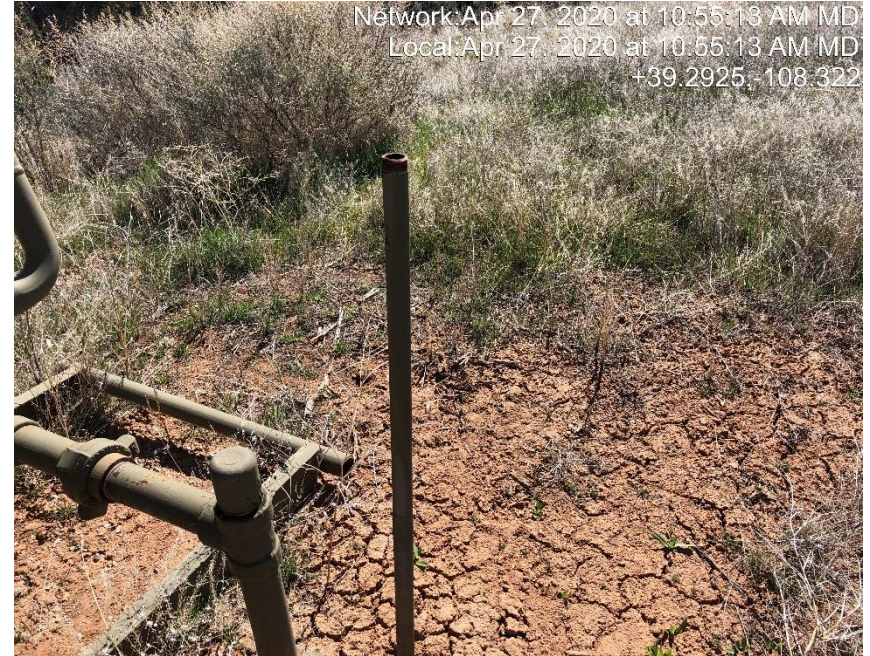
Photo #1049 Flow line riser not LO/TO.
