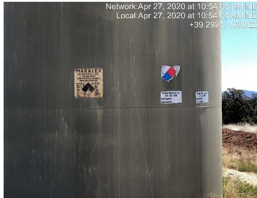
Photo #1046 Tank capacity, contents and NFPA labels weathered and not legible.
