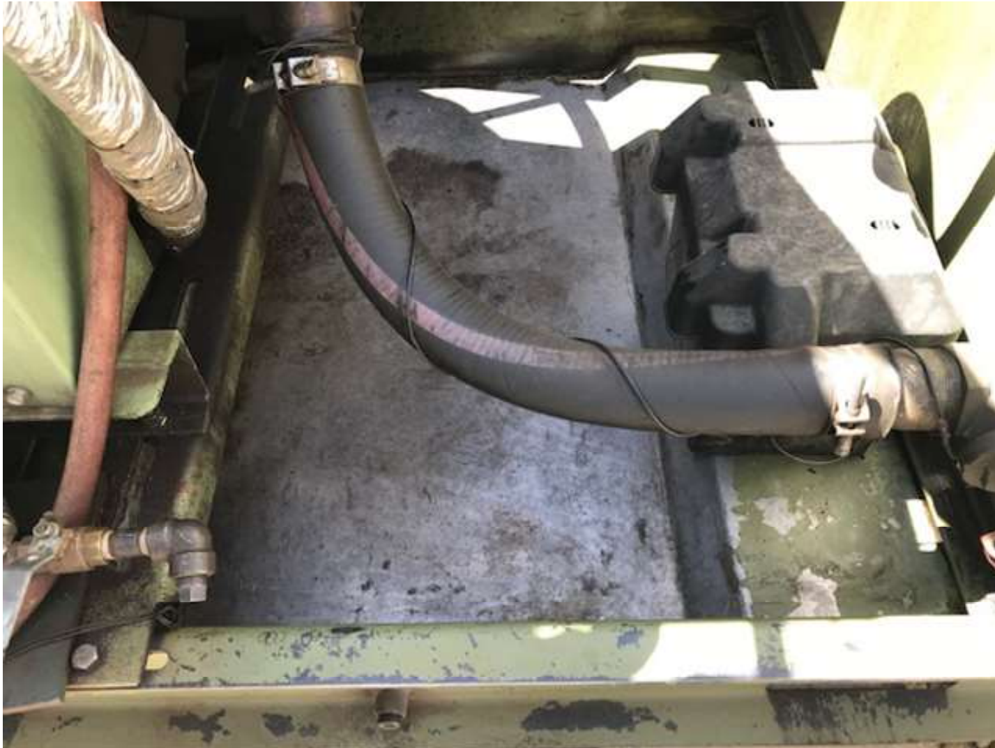
PHOTO 2: THE FLUID ACCUMULATION IN THE ENGINE SKID CONTAINMENT WAS REMOVED AND THE SKID WAS CLEANED UP.
