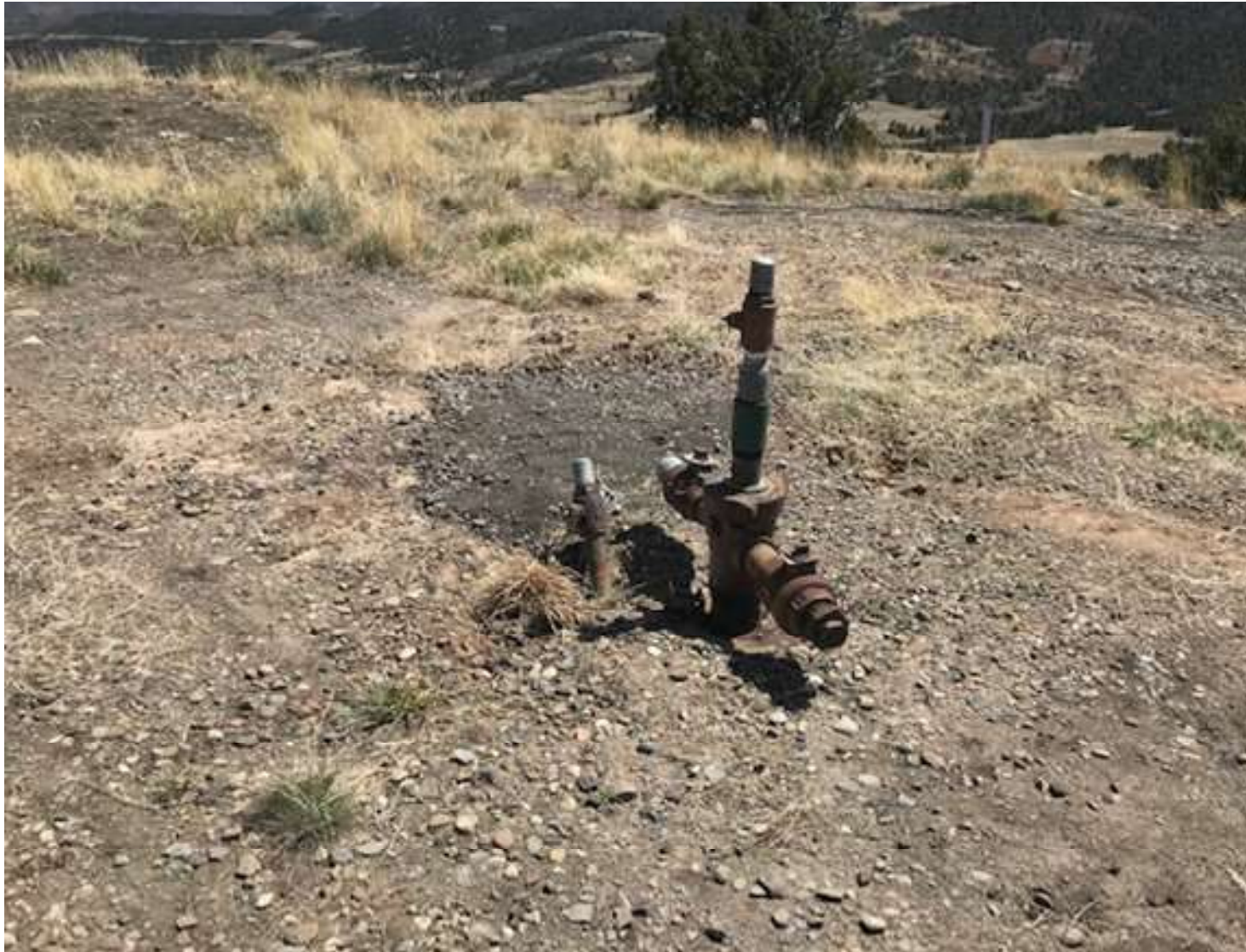
PHOTO 5: THE UNUSED RISERS AT THE GE 28-07X WELLHEAD WERE REMOVED.
