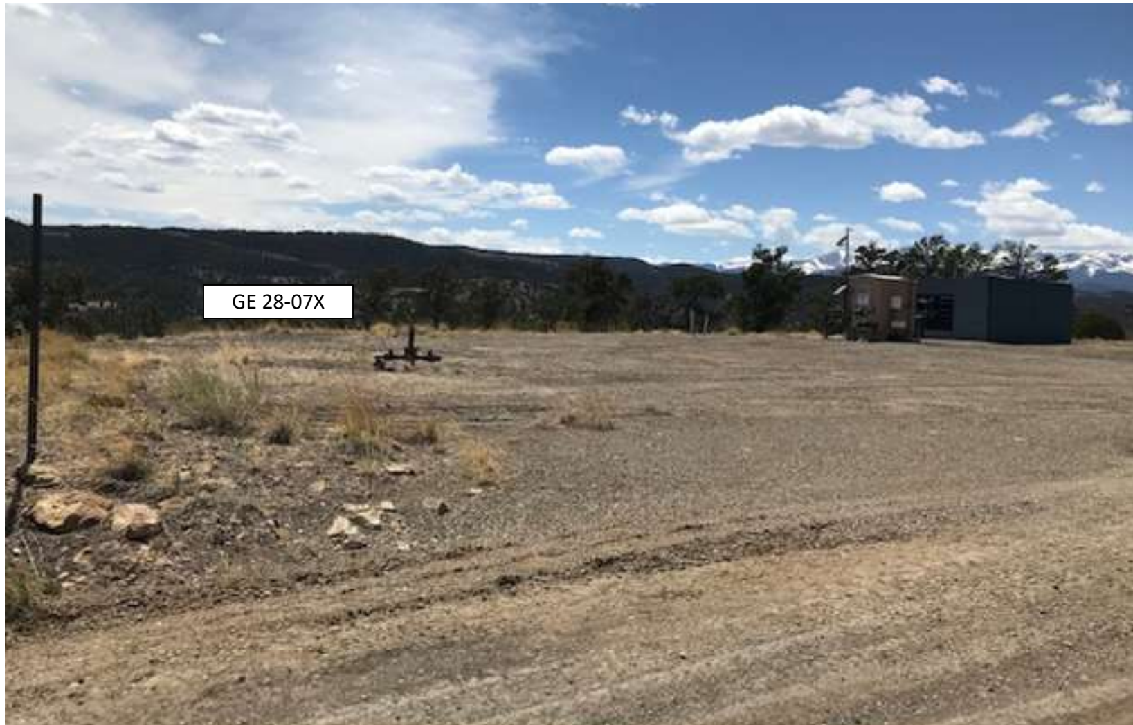
PHOTO 7: THE UNUSED PC ENGINE SKID AND SOUND WALLS AT THE GE 28-07X WERE REMOVED FROM THE LOCATION. THE STAINS ON THE GROUND NEAR PC SKID AND SOUND WALLS HAS BEEN CLEANED UP. (2) RISERS AND THE ABOVE GROUND PRODUCED WATER STORAGE TANK WERE ALSO REMOVED FROM THE LOCATION.
