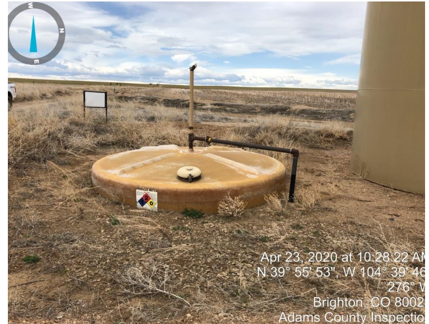
Photo#2 Corrective Action: Amount label missing on pit
