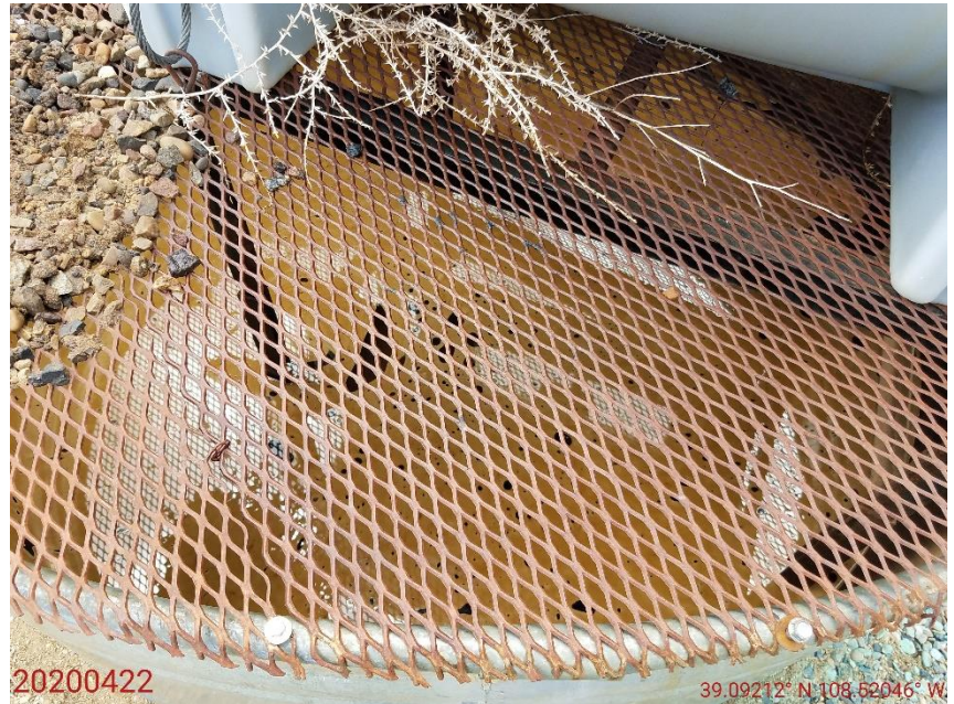
Photo 64: Continued from photo 63. Photo shows chemicals/fluids within secondary containment that needs to be removed.
