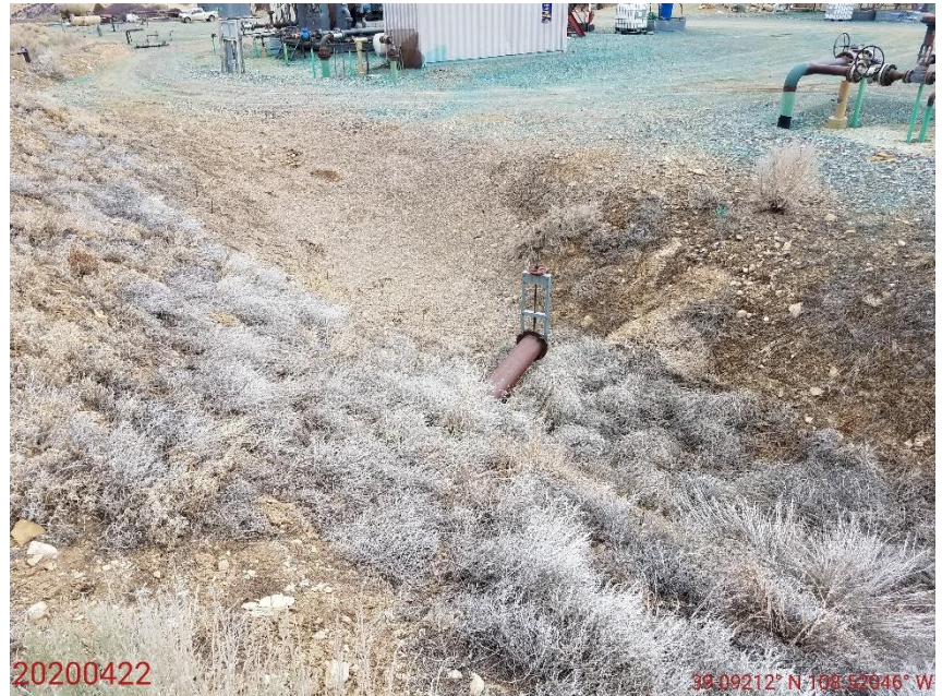
Photo 52: Photo taken from the southwest end of the Location, facing north. Photo shows stormwater containment pond. Pipe with gate installed to allow flow/discharge. Outlet of BMP appears to discharge directly into a creek adjacent to the Location.
