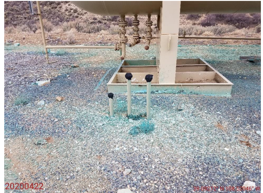
Photo 14: Photo taken from the north end of the Location. Photo shows unused/abandoned equipment (risers) on Location. All unused/abandoned equipment requires removal in accordance with Rule 603.f
