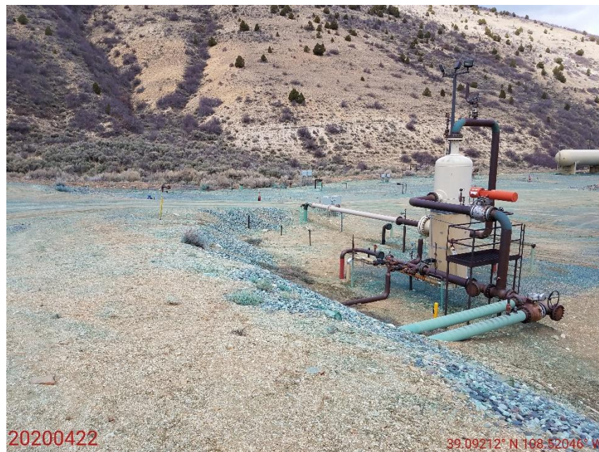
Photo 66: Photo taken from the east end of the Location, facing northwest. Photo shows vertical separator that appears to remain in use on Location.
