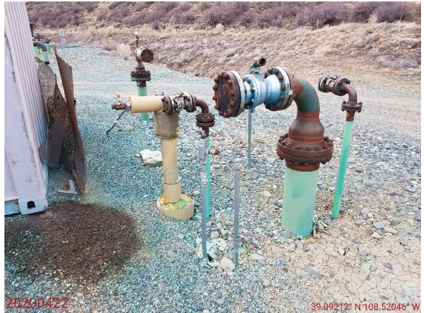
Photo 42: Photo taken from the north end of the Location, facing southwest. Photo shows unused/abandoned equipment (risers) on Location. Equipment appears to have been associated with a compressor, that has since been removed. All unused/abandoned equipment requires removal in accordance with Rule 603.f. Photo also shows stained soils.
