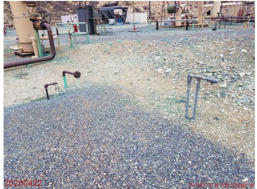
Photo 62: Photo taken from the east end of the Location, facing northwest. Photo shows unused/abandoned equipment (risers) on Location. All unused/abandoned equipment requires removal in accordance with Rule 603.f.
