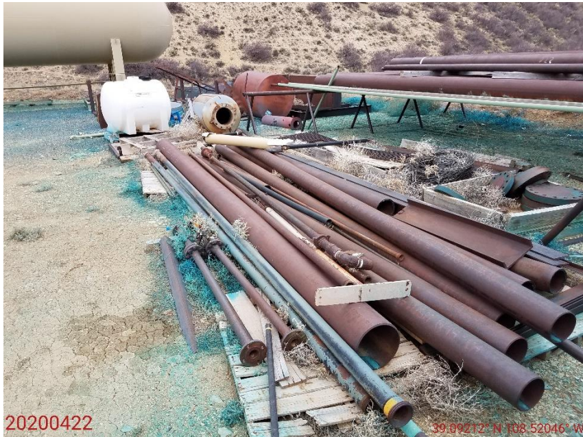
Photo 11: Photo taken from the north end of the Location. Photo shows unused equipment (pipe, tanks, etc...) and trash debris stored on Location. All stored/unused equipment and trash debris requires removal in accordance with Rule 603.f
