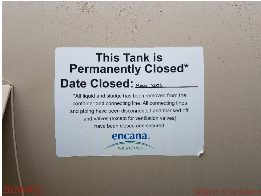
Photo 13: Photo of sign on tank observed in photo 12. Photo shows tank has been “permanently closed” since March 2006. Tank is considered unused equipment and requires removal.
