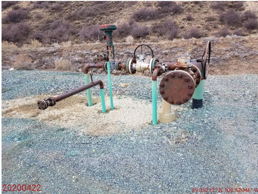
Photo 47: Photo taken from the southwest area of the Location. Photo shows unused/abandoned equipment (risers) on Location. Equipment appears to have been associated with a compressor, that has since been removed. All unused/abandoned equipment requires removal in accordance with Rule 603.f. Photo also shows stained soils.
