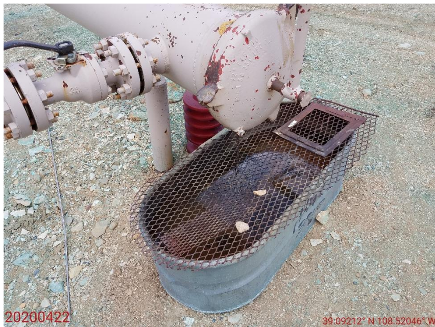
Photo 65: Photo taken from east end of the Location. Photo shows chemicals/fluids within secondary containment that needs to be removed.
