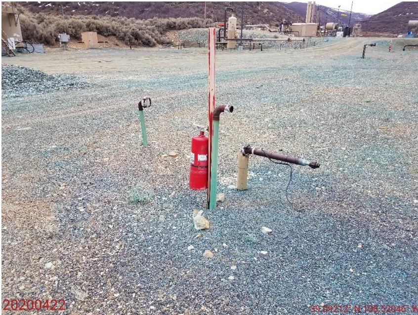
Photo 19: Photo taken from the northwest end of the Location, facing southeast. Photo shows unused/abandoned equipment (risers) on Location. All unused/abandoned equipment requires removal in accordance with Rule 603.f
