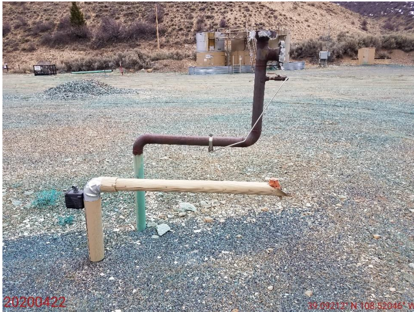
Photo 21: Photo taken from the northwest end of the Location, facing east. Photo shows unused/abandoned equipment (risers) on Location. Equipment appears to have been associated with a compressor, that has since been removed. All unused/abandoned equipment requires removal in accordance with Rule 603.f
