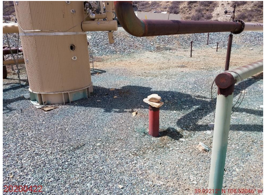
Photo 68: Photo taken from the northeast end of the vertical separator. Photo shows unused/abandoned equipment (risers) on Location, with stones placed upon the open pipe; this is improper capping procedure. All unused/abandoned equipment requires removal in accordance with Rule 603.f.
