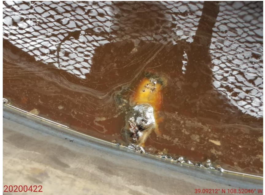
Photo 46: Continued from photo 45. Photo shows containment BMP has filled with chemicals/fluids. Photo also shows wildlife appears to have entered and died within the BMP.
