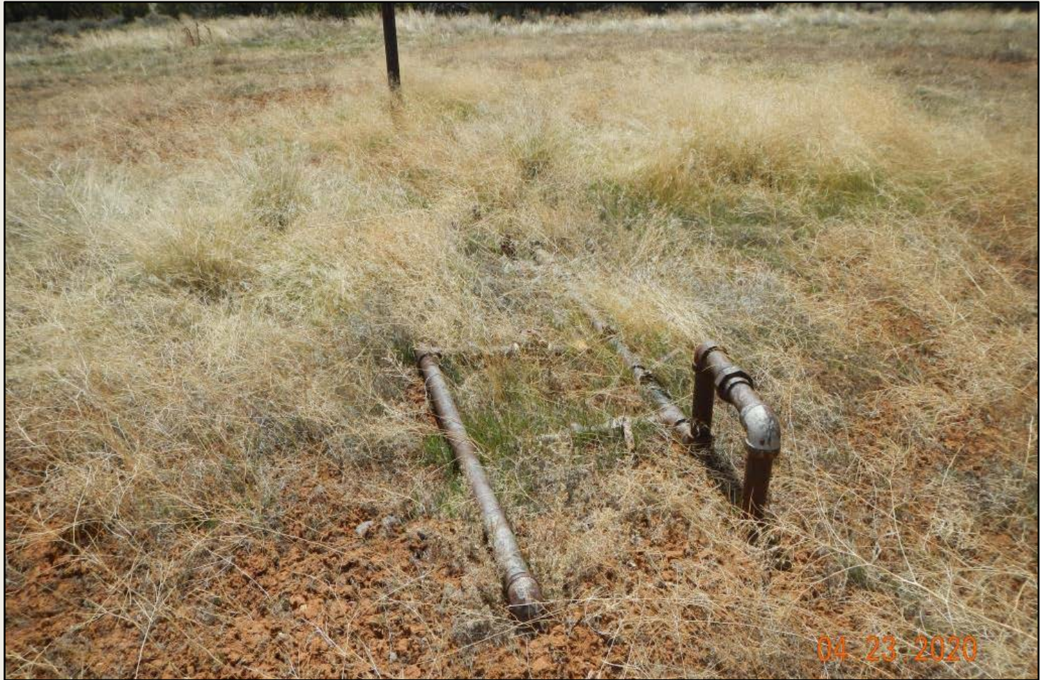
Photo 5. View of plugged well marker and remaining lines around plugged well location.
