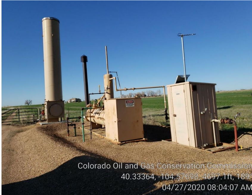
Photo #3 Separator, ECD & Meter Run
