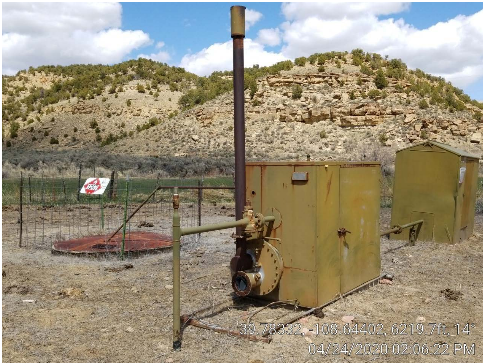
Photo 2. Pit, separator, meter building.
