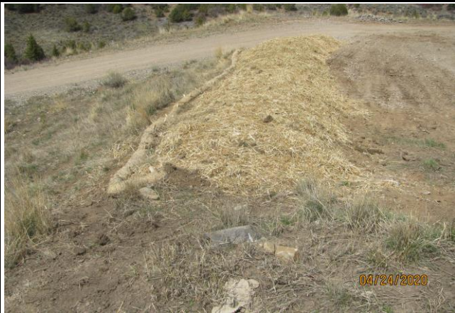
BMPs Installed on the Berm South of the Entrance on the Hells Gulch 26-06 Pad
