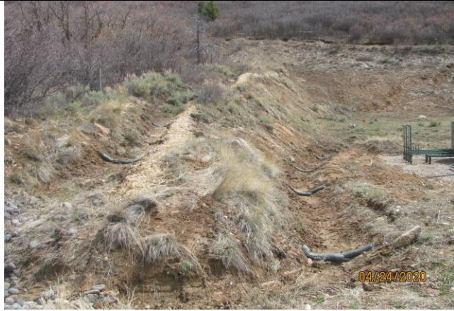
Drainage Ditch Repaired on the East Side of the Hells Gulch 26-06 Pad
