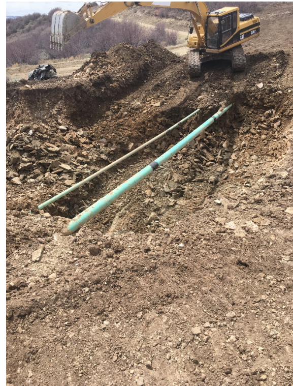
photo at time of inspection 4" replacing 10"
