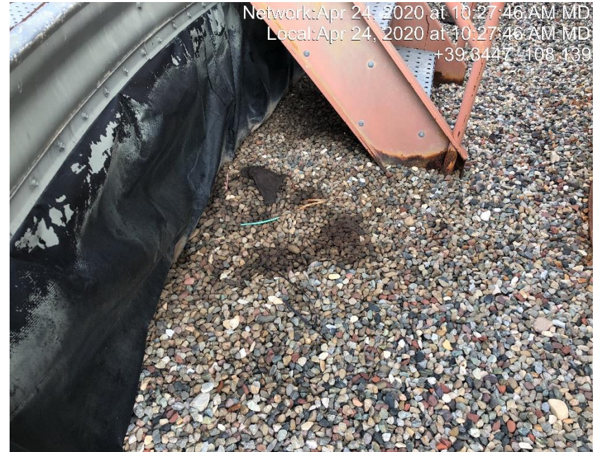
Photo #1037 Stained gravel inside tank containment.
