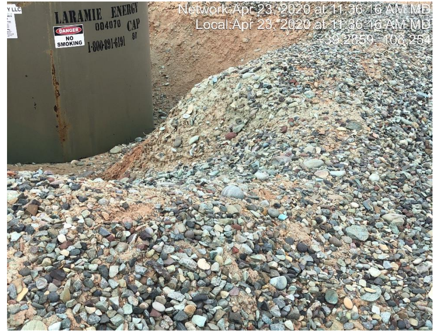
Photo #1028 Secondary containment berm has eroded.
