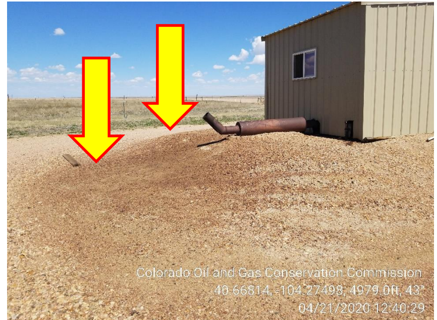
Photo 6 – Stained Soil at Exhaust
