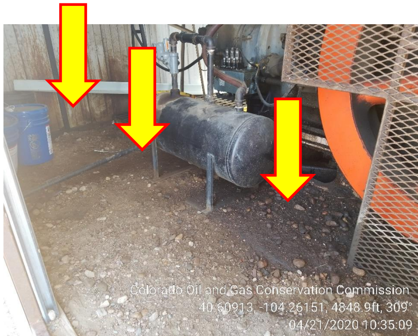
Photo 5 – Stained Soil inside the Engine Housing
