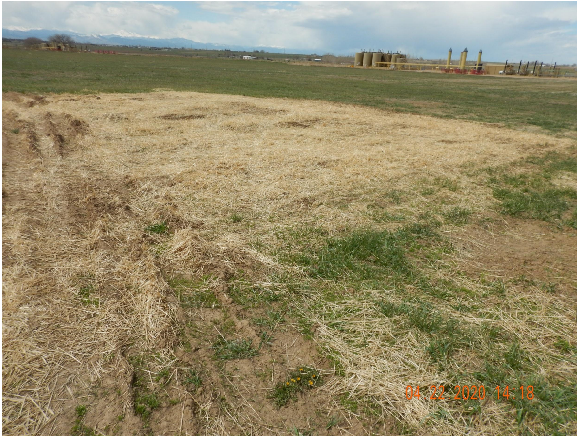
Photo 1. Photo taken from the well location, facing West. Photo illustrates Operator performed final reclamation activities with the evidence of drill rows and straw crimped mulch.
