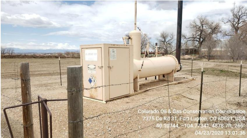
**Photo 7 Horizontal Heated Separator**
