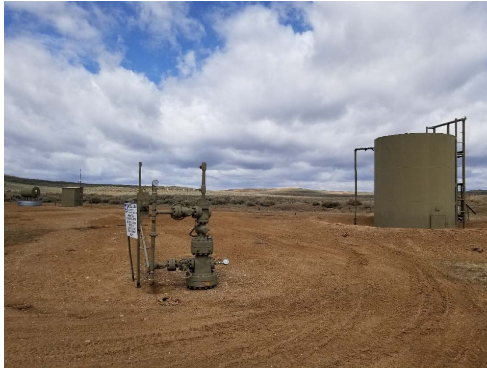
Photo 1. Overview of location taken facing south.
