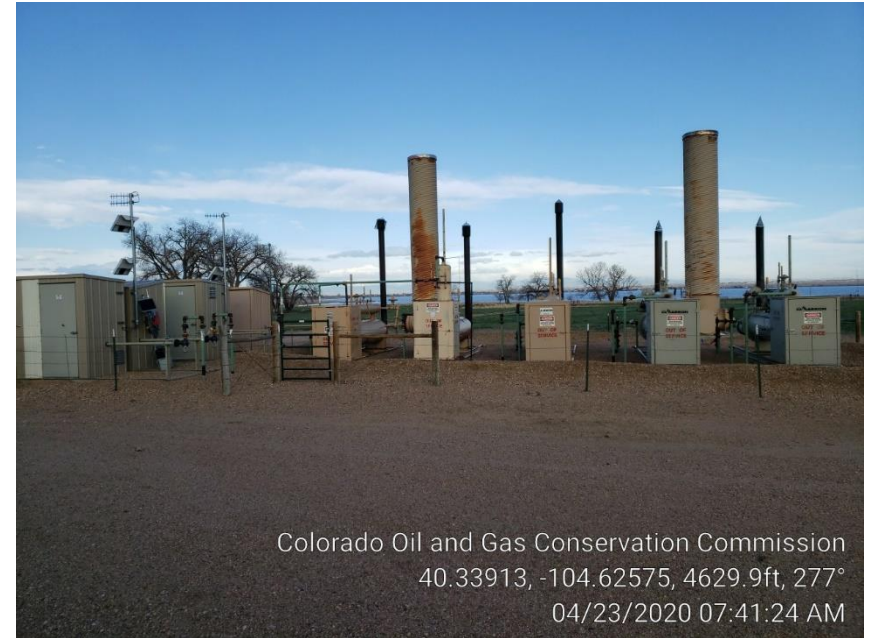
Photo #11 Separators, ECD's & Meter Runs
