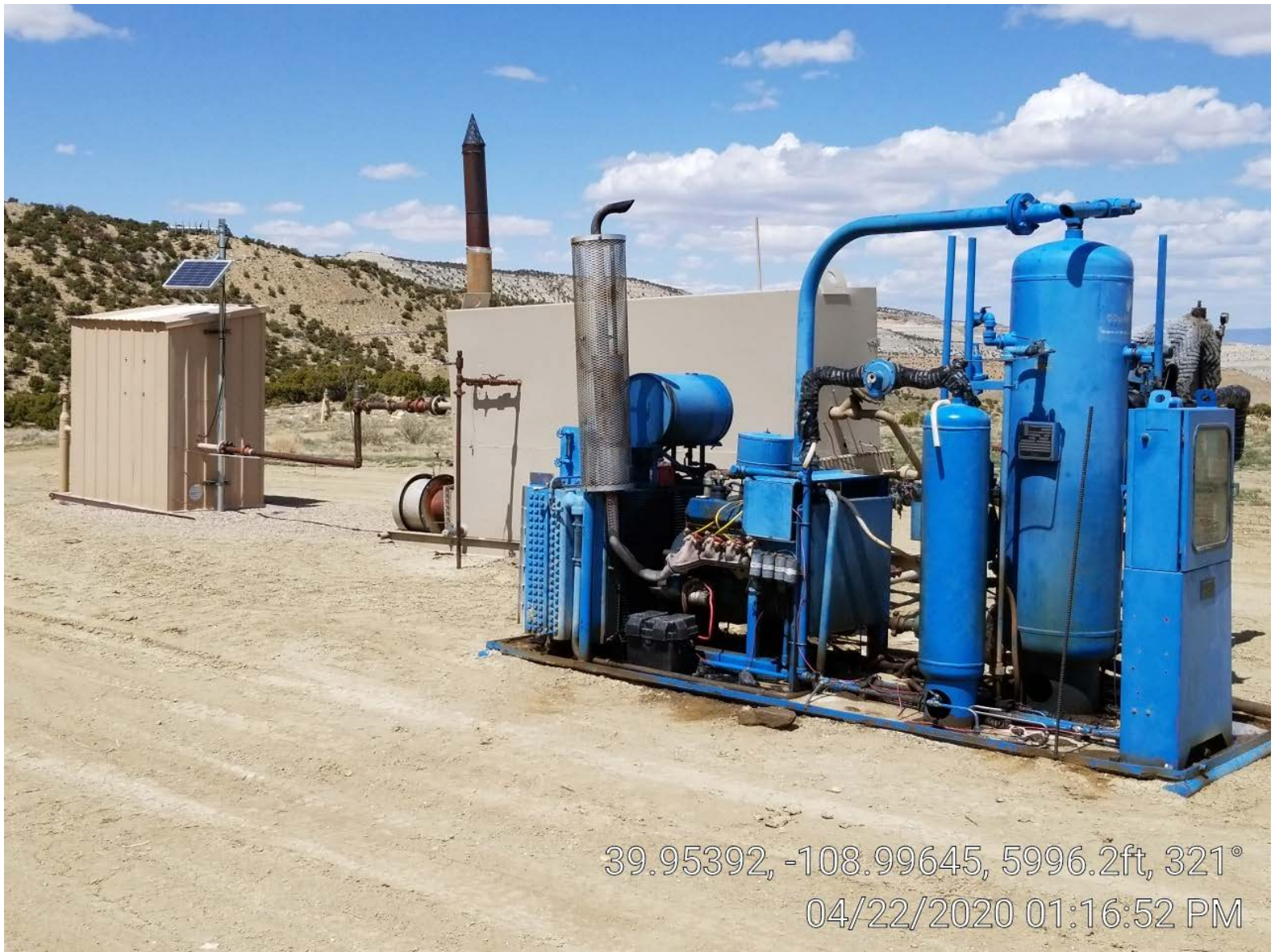
Photo 3. Meter building, separator, and compressor.
