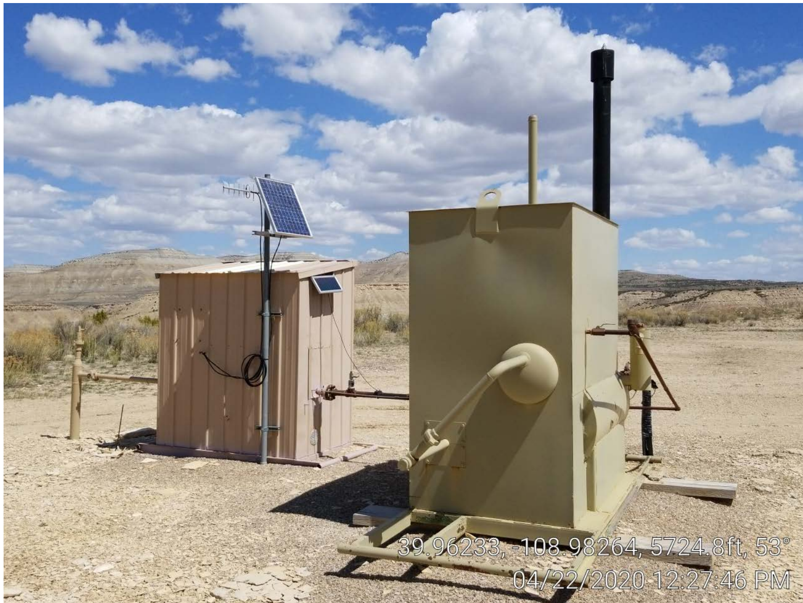
Photo 2. Meter building & separator.
