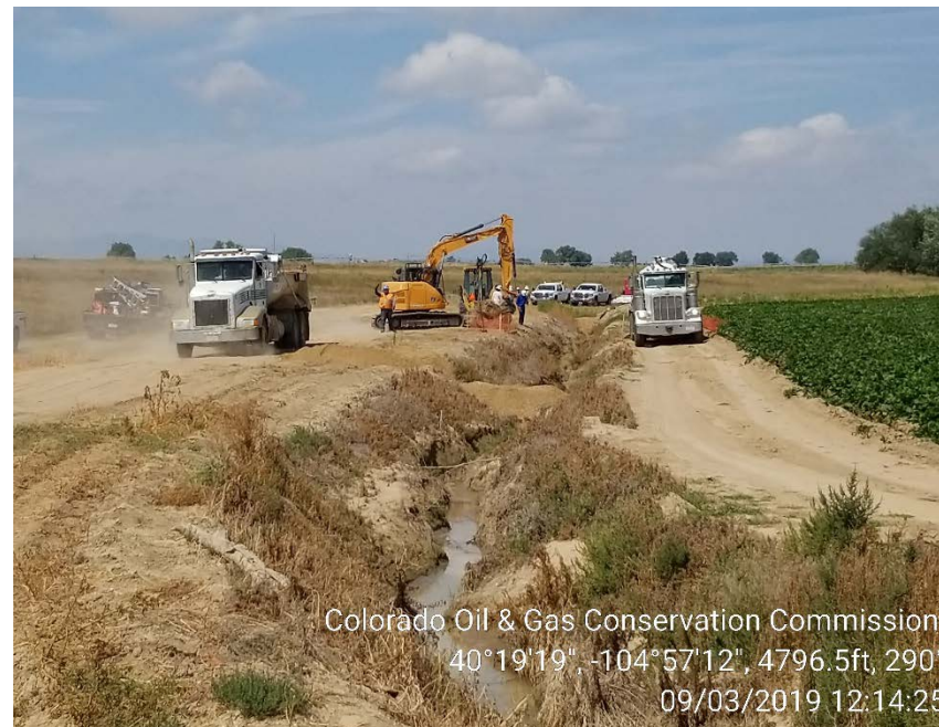
Excavation to expose the release point.
