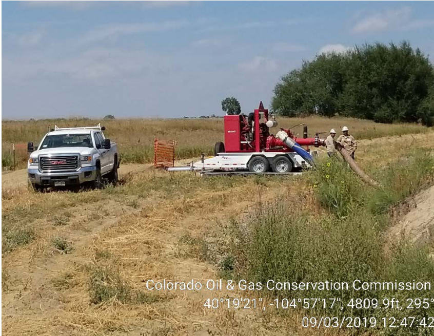
Pumping to manage water above the temporary dam.
