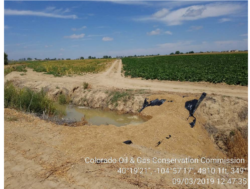
Temporary dam in the ditch.
