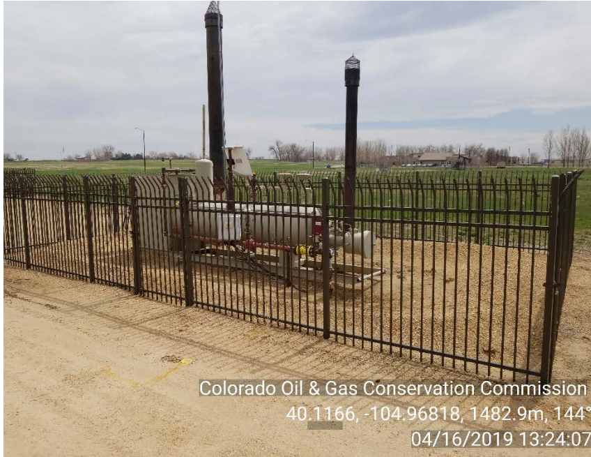
Photo 3: Horizontal Separator
