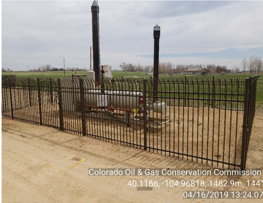
Photo 3: Horizontal Separator
