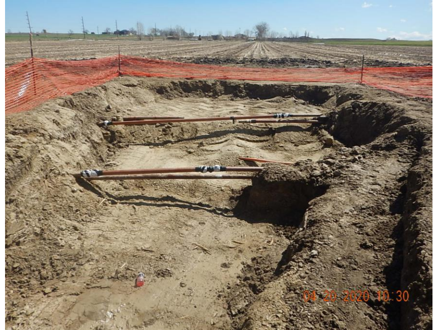
View of excavation and flowlines exposed (to east)
