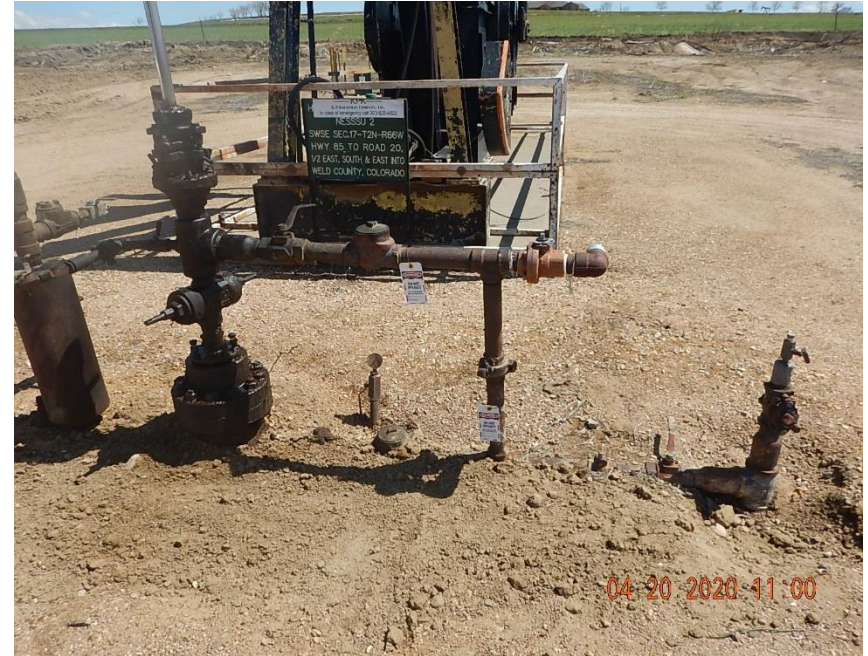
View of Nessu #2 wellhead (API 123-08811); OOSLAT (flowline shut in/ tagged out)
