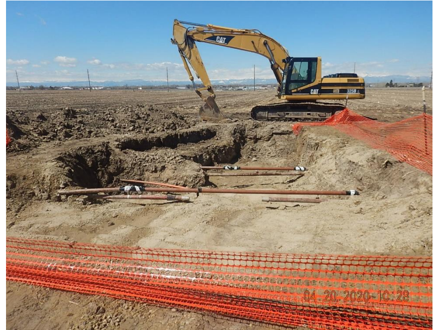
Closer view of excavation at Spill ID # 470915 with flowlines exposed (looking West)
