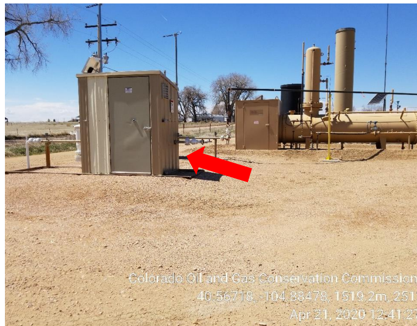
Photo 6: Equipment removed; DISCONNECTED/UNUSED GAS METER
