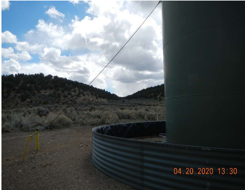
Tank battery secondary containment and guy line anchor
