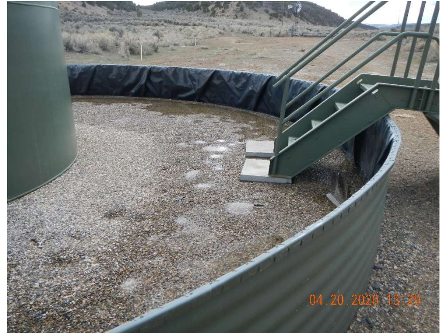
Tank battery secondary containment and stormwater
