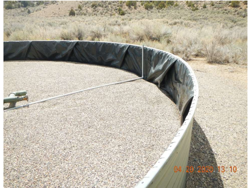
Tank battery secondary containment
