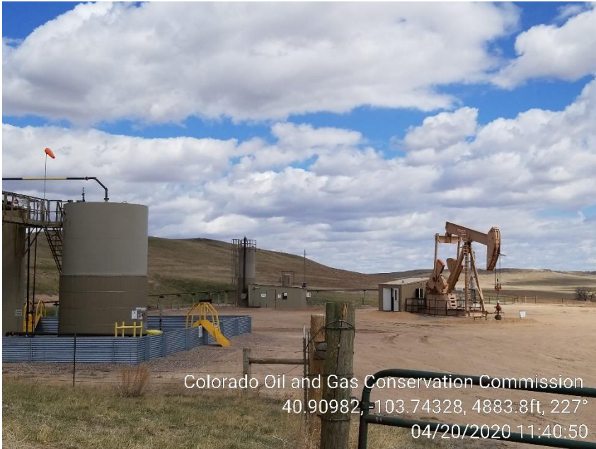
Photo 1 – Tank Battery
