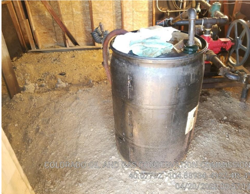
Pic 3 no BMP under barrel in pump house
