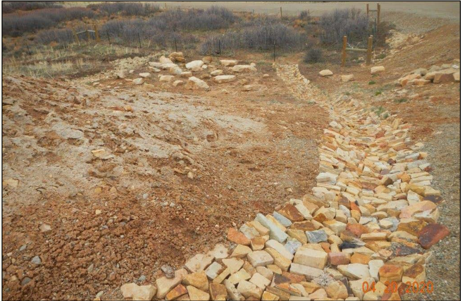
Photo 4. View of course rock run-down at well pad entrance appears to be functioning at this time.
