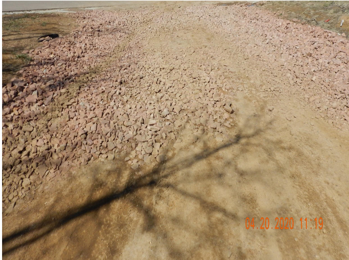
Photo 4. Photo taken from the entrance of location, facing West. Photo illustrates the vehicle tracking device BMP is in need of maintenance.
