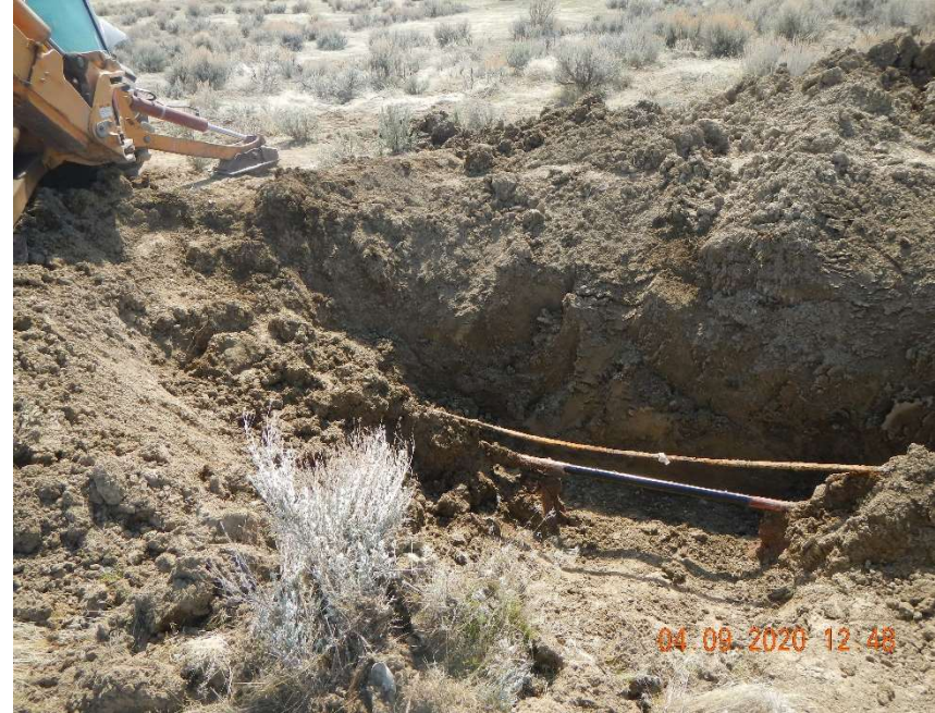
Excavation, repaired flowline and electrical conduit.
