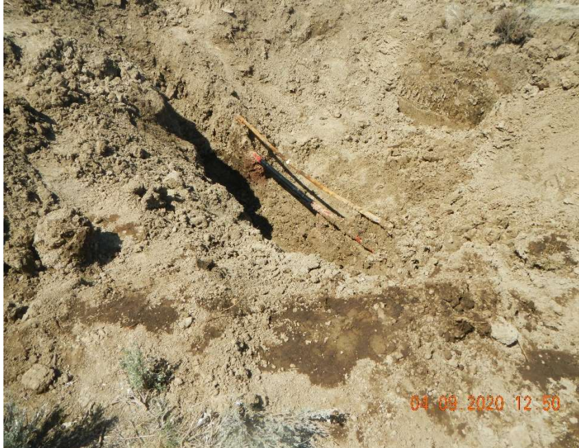
Excavation, impacted material from the excavation, repaired flowline and electrical conduit.
