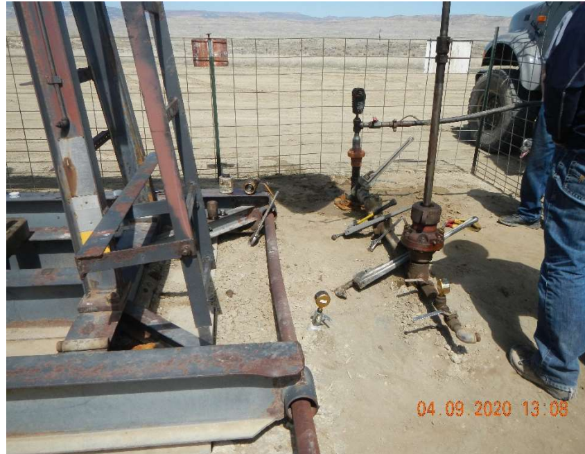
Pressure testing the repaired flowline with water.
